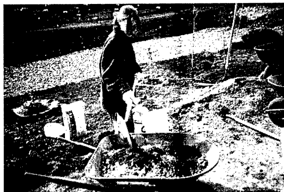
Figure 13. Dredged material added
