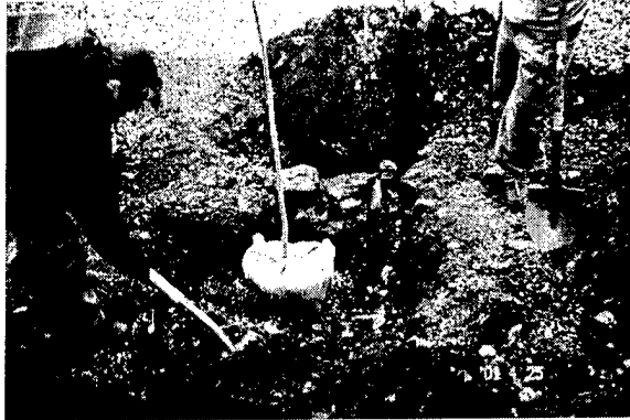
Figure 15. RSMT blend being placed in hole under tree root ball
