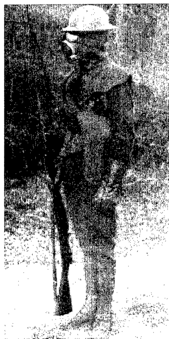
Fig. 2-26. In addition to the standard Service Gas Mask, the Chemical Warfare Service also designed diaphragm masks for speaking capability. Note the hood, which covered the skin of the head, face, and neck. The soldier also wears chemically protective gloves. Since the uniform was impregnated with a substance that hindered the penetration of mustard, in theory, no portion of his skin was subject to mustard injury. Photograph: Chemical and Biological Defense Command Historical Research and Response Team, Aberdeen Proving Ground, Md.
