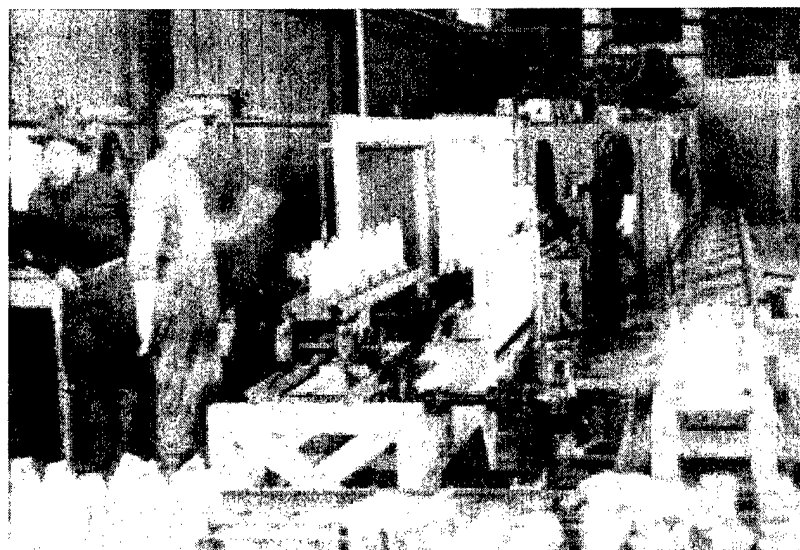
Fig. 2-7. Filling 75-mm artillery shells with mustard agent at Edgewood Arsenal, Md. Facilities designed to fill shells with chemical agents were notoriously hazardous. Anecdotal reports from mustard shell-filling plants indicated that over several months, the entire labor force could be expected to become ill. These workers' apparent nonchalance to the hazards of mustard would not be tolerated by the occupational medicine standards of a later era (see Figure 2-31). Photograph: Chemical and Biological Defense Command Historical Research and Response Team, Aberdeen Proving Ground, Md.
