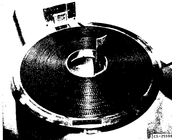
FIGURE 49-6.—Liquid-neon-cooled coil.
