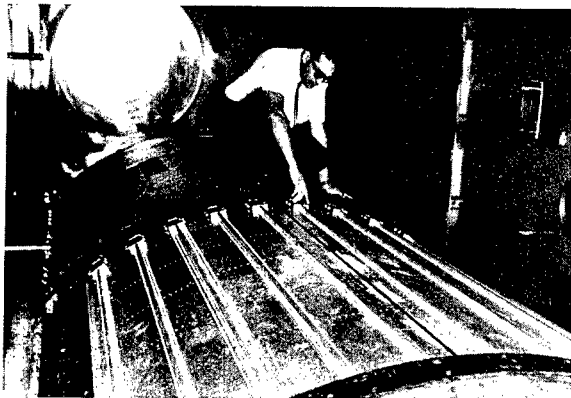
FIGURE 72-7.—Launch-vehicle interstage structure.
