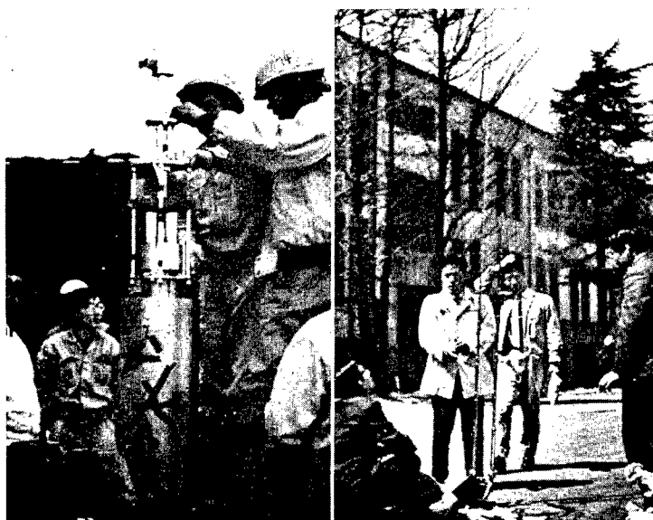
Nosecone opening function test: from top are geomagnetic aspect meter, RN loop antenna, and cosmic-ray counter.
