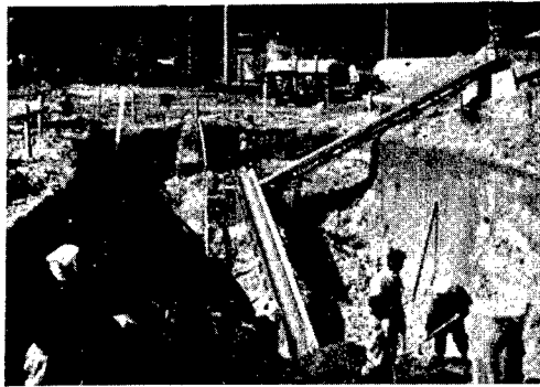
Fig. 6. Work to dig flame channel for rocket-transport track
