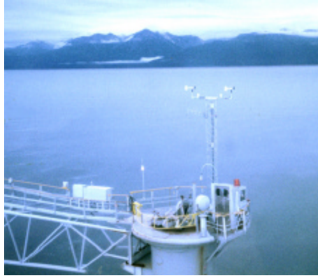
Figure 2. Weather monitoring in difficult places. This fixed sensor was installed on an offshore platform 90 miles Southwest of Anchorage, Alaska on 31 Aug 1999. Photo: courtesy of NOAA.
