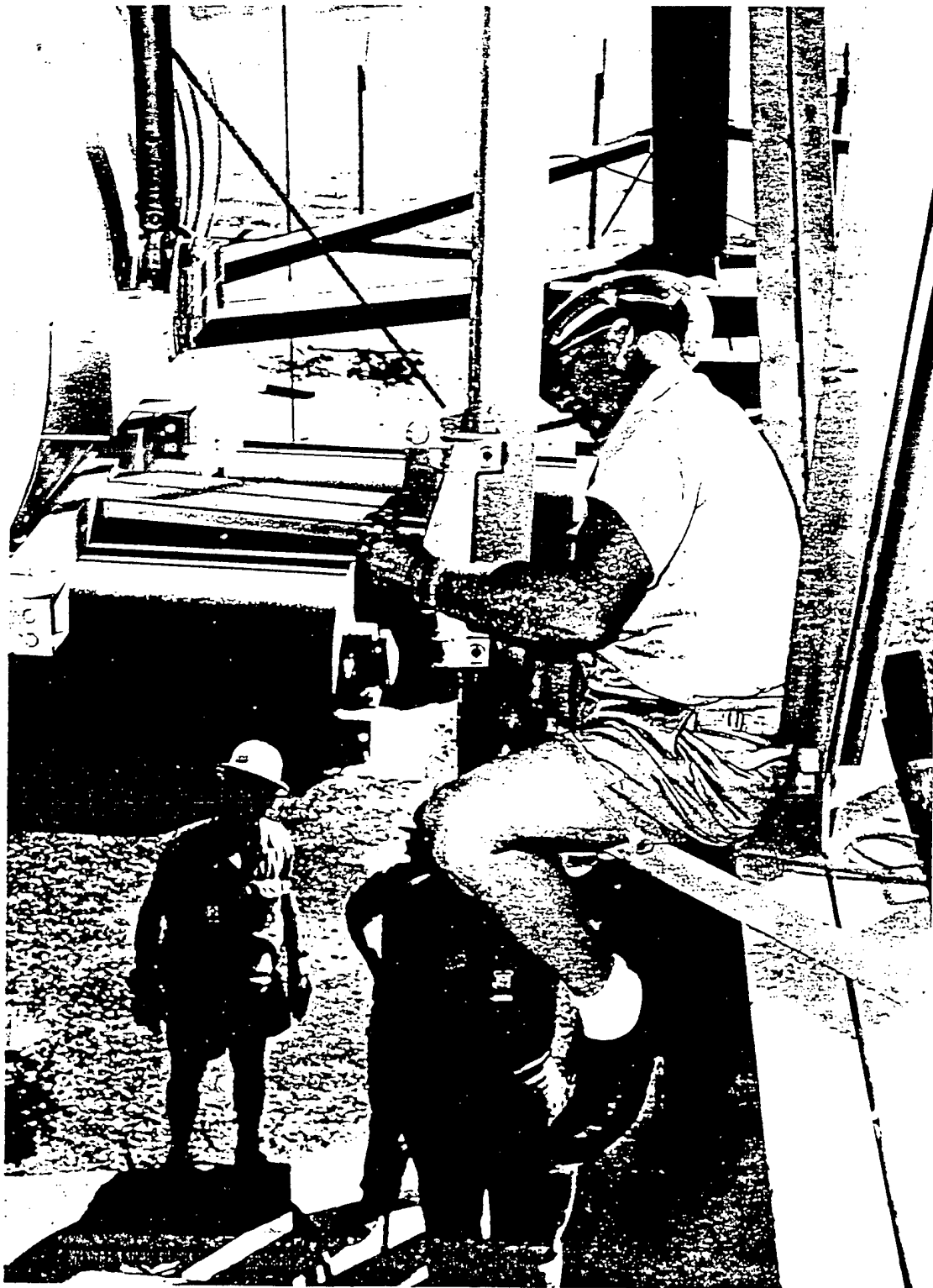
Fig. 3.32 Engaging Roller Skates on Guide Rails
