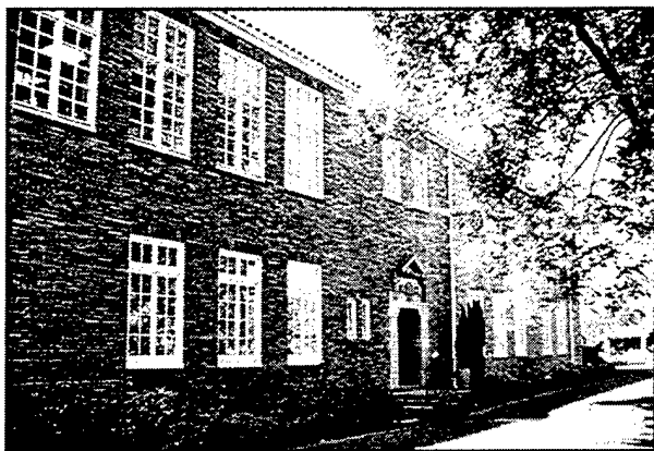
Figure 46. Exterior view of the Jones and Stokes repository.
