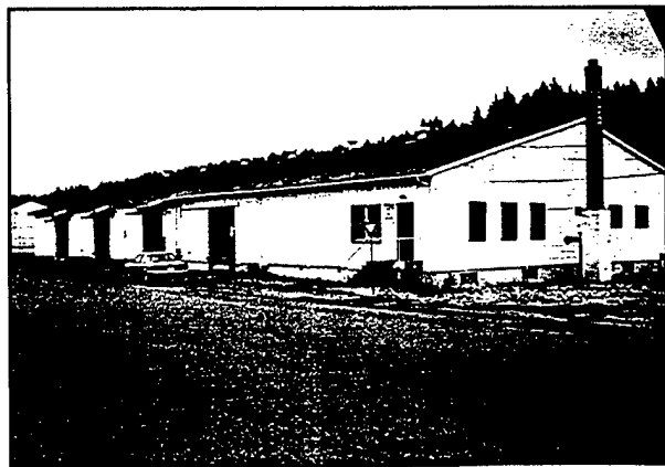
Figure 2. Front view of Forestry Supply Repository (Building T1214) at Fort Lewis.
