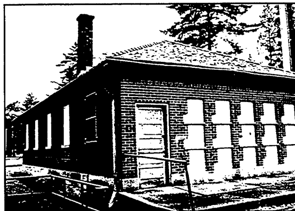
Figure 3. View of Veterinary Building (T4294) at Fort Lewis.
