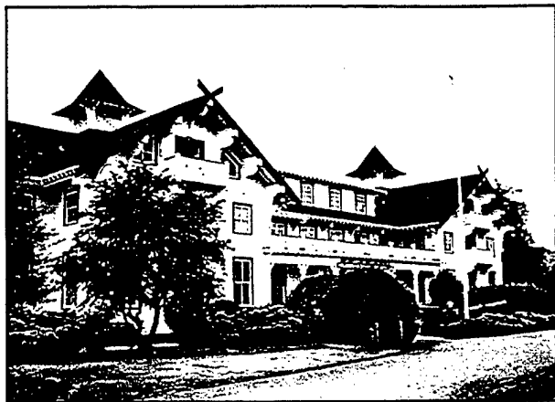
Figure 1. Exterior view of the Fort Lewis Military Museum.
