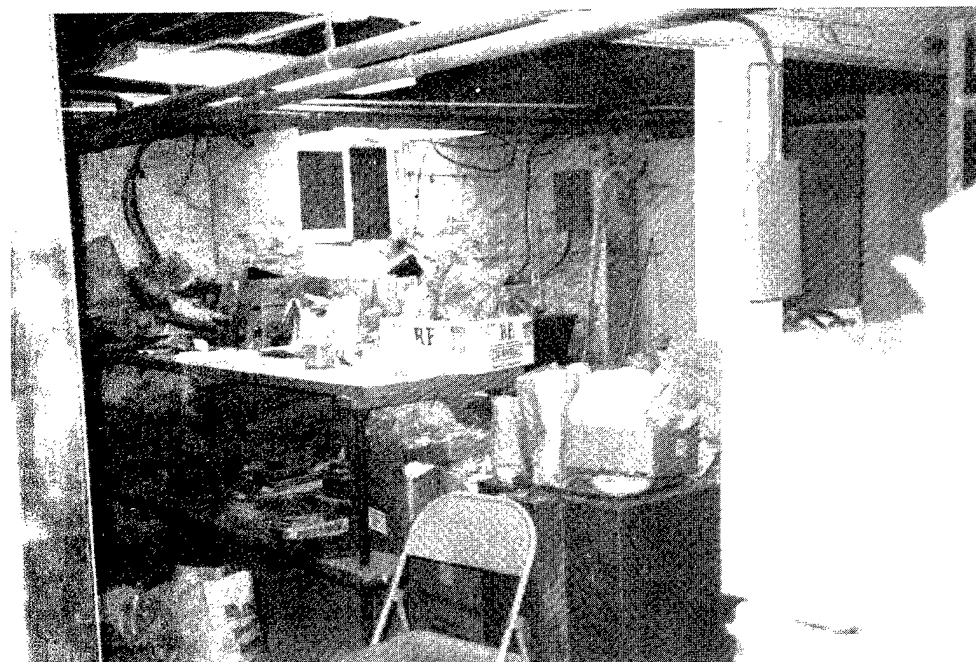
Figure 6: Cluttered storage areas, exposed wiring, and overhead water pipes endanger collections.
