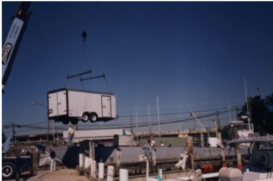
Figure 3. Loading on LCM-8 for Chesapeake tests.
