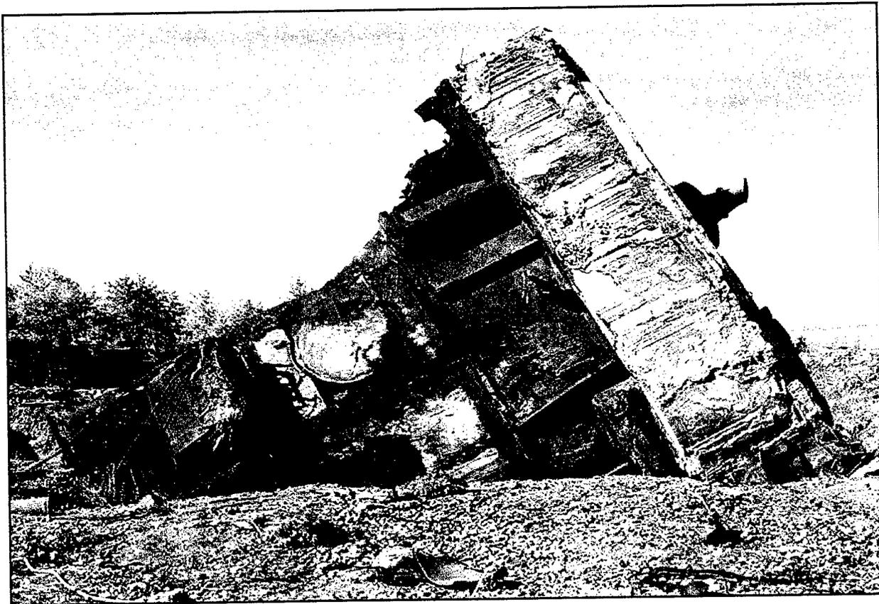
Figure 37. Relatively intact LCC silo door pocket still attached to part of the headworks wall.
