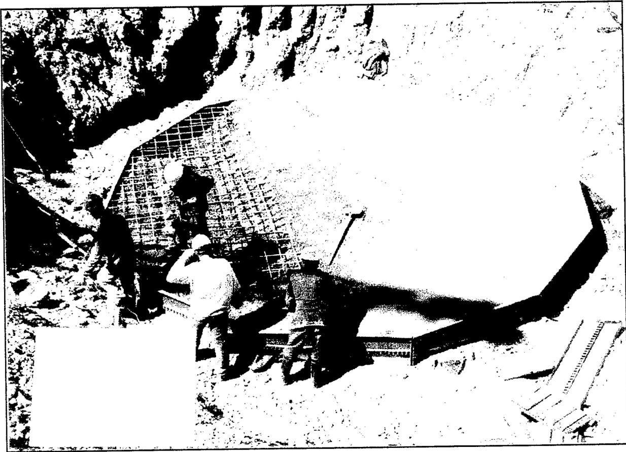
Figure 41. Pouring the eight meter diameter reinforced concrete cap over the filled silo tube.
