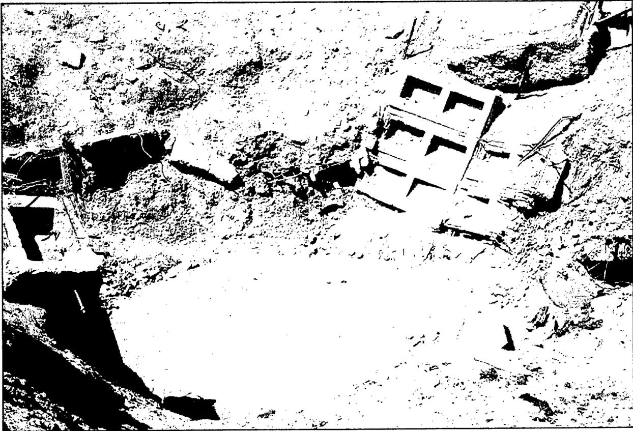
Figure 42. Poured reinforced concrete cap in place over the filled silo tube. Part of the "barbette" wall is exposed in the crater. Derzhavinsk, Regiment 3, Silos 5/7.
