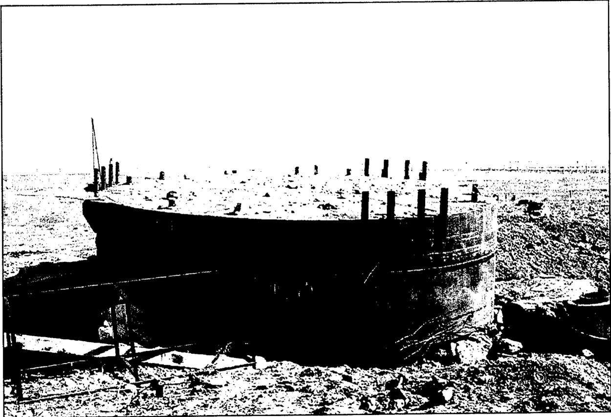
Figure 14. Round silo door for the Launch Control Center (LCC) silo. Note the difference between this door and the door for a launch silo (compare to Figure 12).
