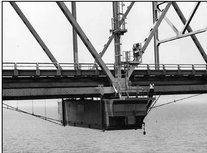
NRL researchers conducted submarine detection experiments from this gondola laboratory suspended below the Chesapeake Bay Bridge.
