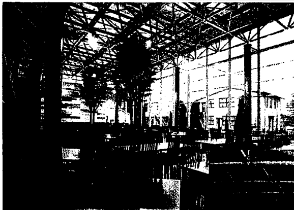
Photo 1: < The Refreshment Room of Toray Industries Factory in Ehime > Roof Area: 350 m 2 Total Construction Terms: March 1997 ~ September 1997
