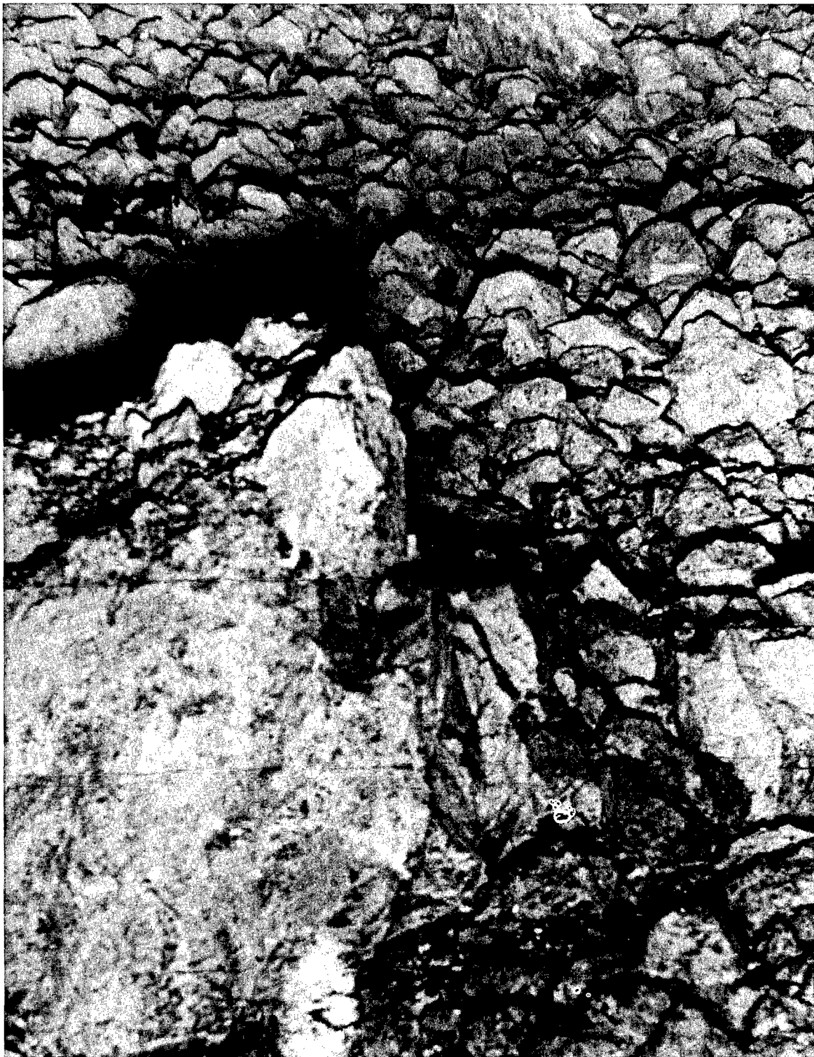
Fig. 5. Top of fragmented rubble in Handcar chimney (dolomite). Large block in foreground has maximum dimension of about 3 ft.
