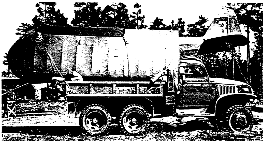
Fig 8. L-4 loaded in a 2 1/2 Ton short bed truck. Source: "Organic Air Observation," Field Artillery Journal 32 (July 1942): 501.
