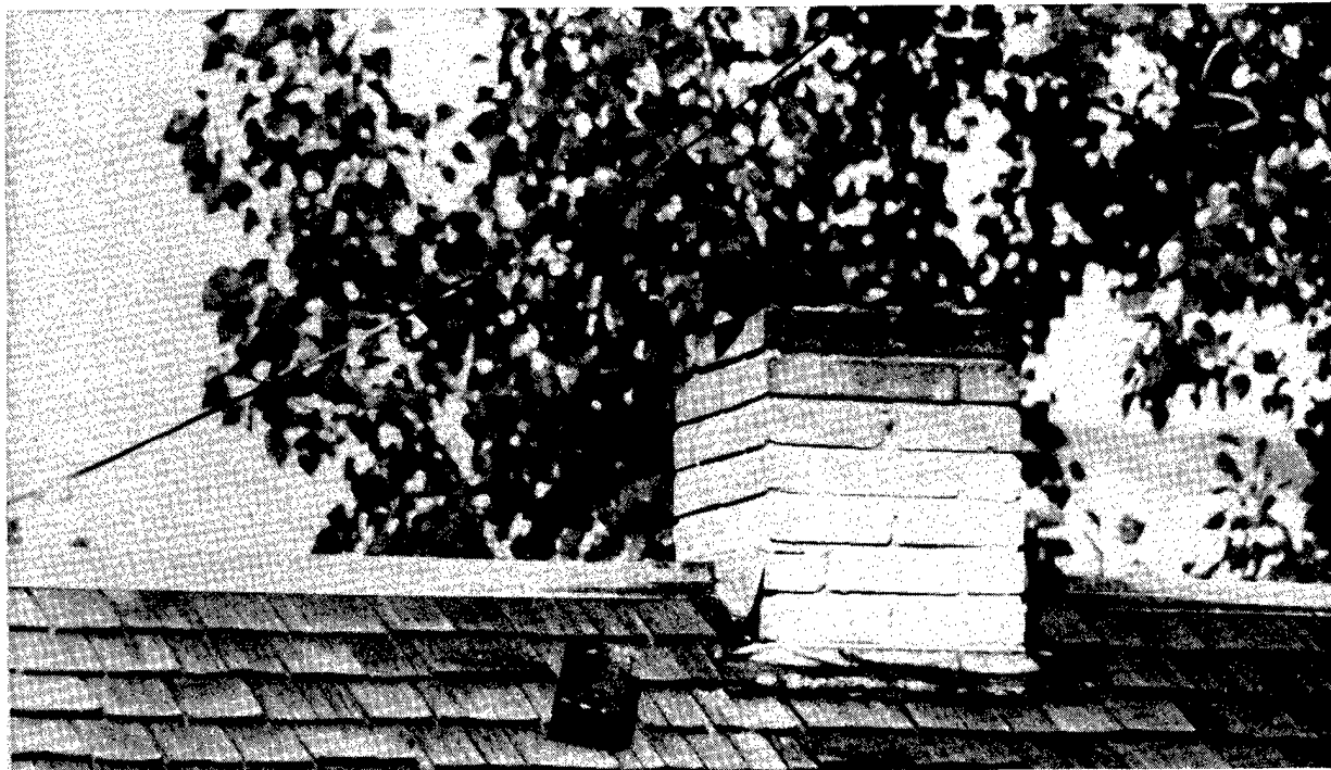
Fig. 10. Example of Rulison damage.
