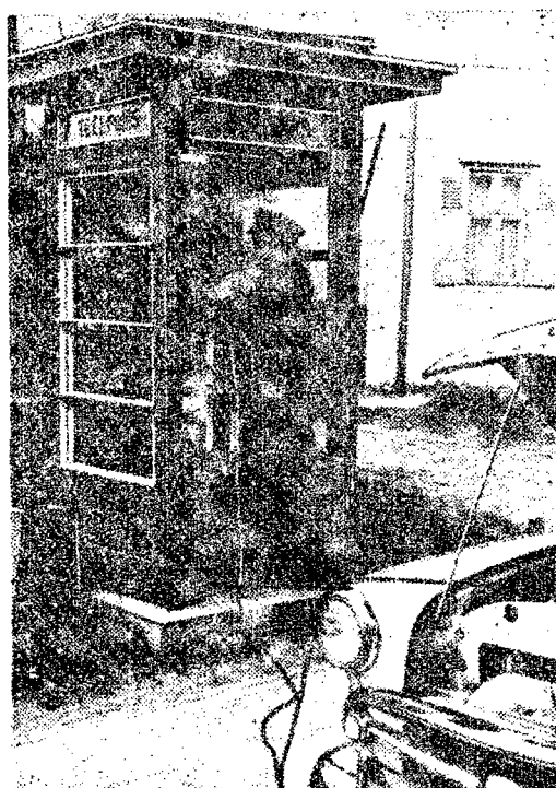
Supervisor A. Ya. Druba repairs a telephone— solders a broken wire with the aid of a special soldering gun connected to the battery of the "Moskvich" car.
