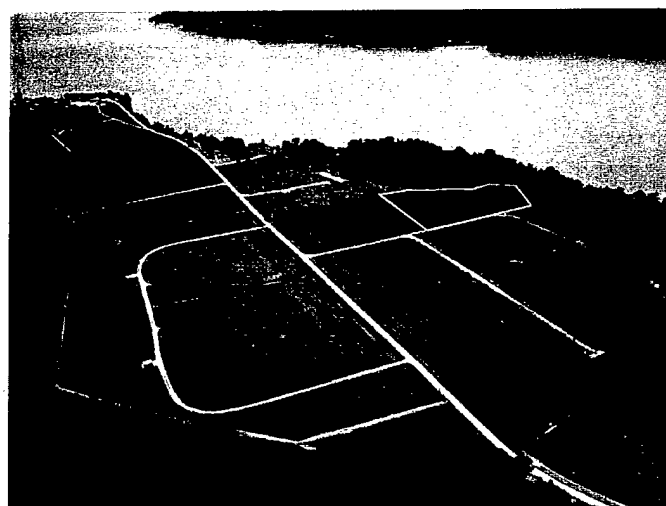
Figure 1. Aerial photograph of the Army Research Lab Facility at Blossom Point, MD. The MTADS Prove Out Test Field is in the area shown outlined in yellow.
