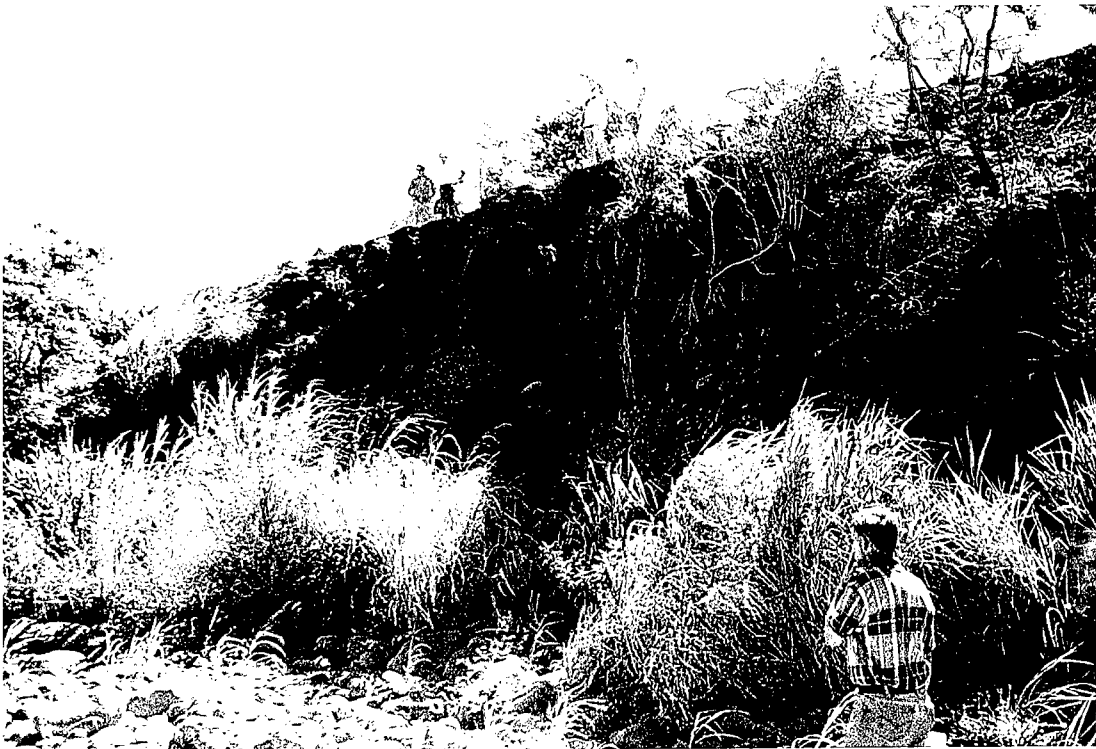
Photo 8. Bank oversteepening due to toe erosion at Sta 40+00
