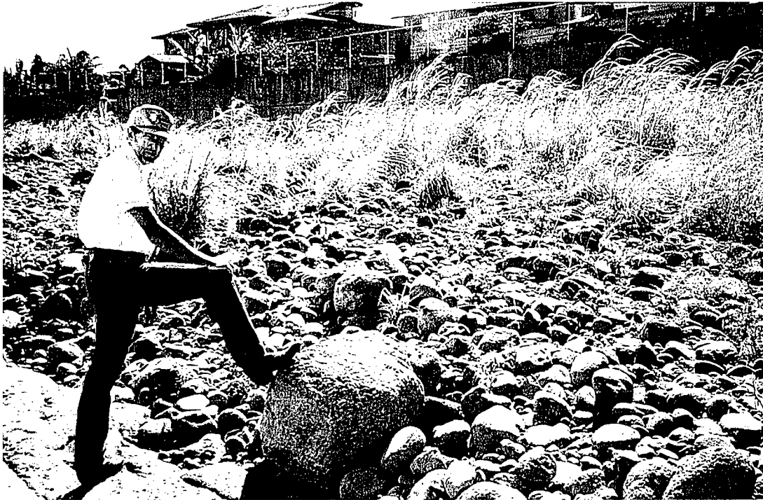
Photo 9. Deposition in boulder-concrete channel downstream from Waiehu Beach Road
