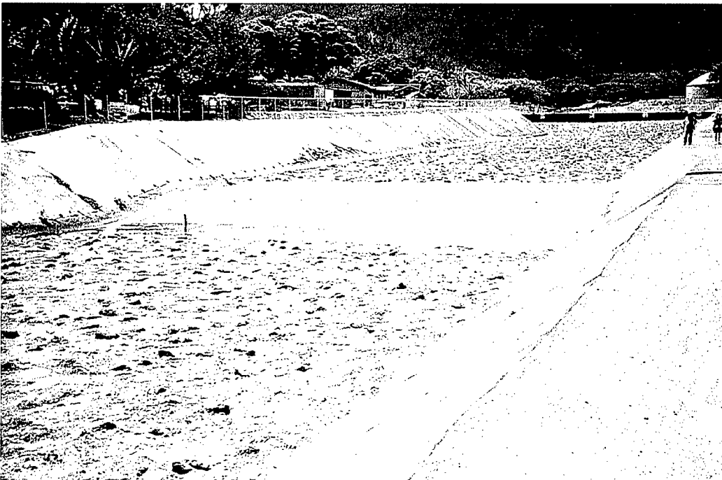
Photo 2. Boulder-concrete channel downstream from sediment basin
