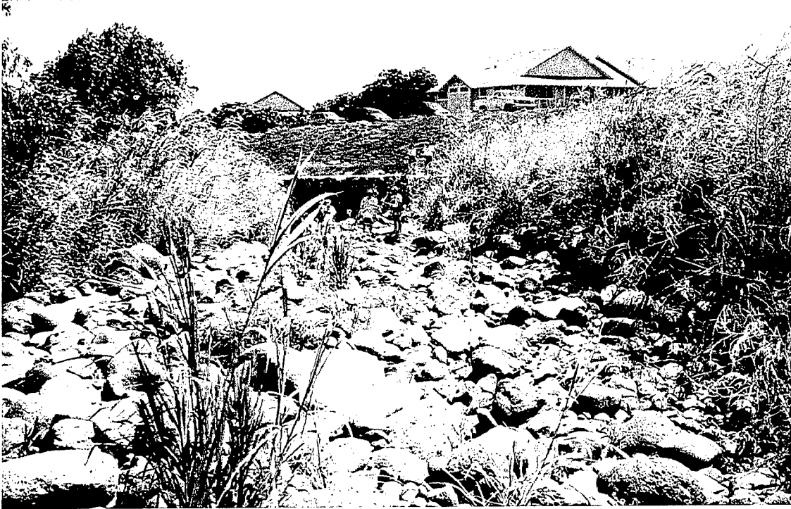
Photo 3. Channel impingement at Sta 50+00
