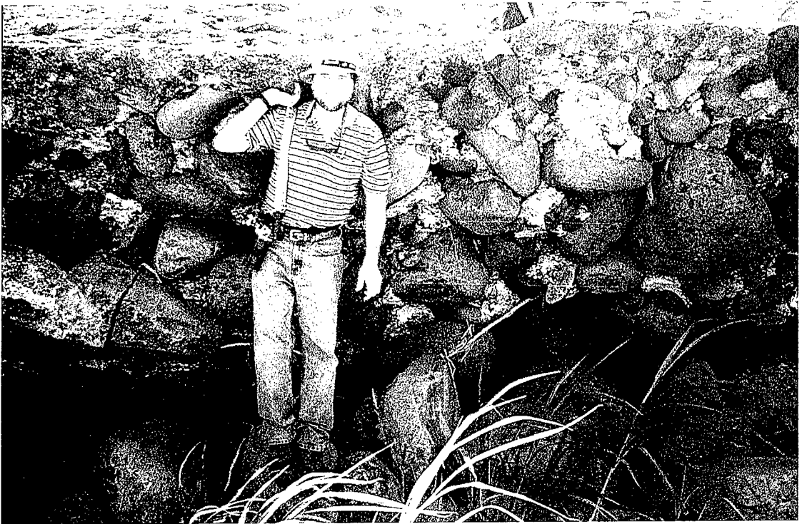
Photo 4. Local scour under grouted stone apron Sta 41+00 to 49+00
