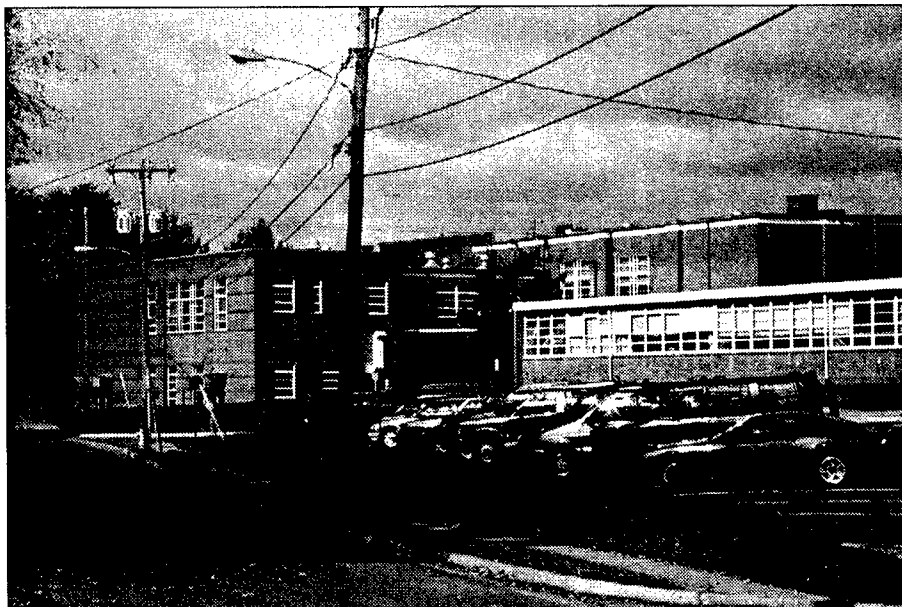
Figure 34. Exterior view of FCAS, which is located in the left portion of this building.
