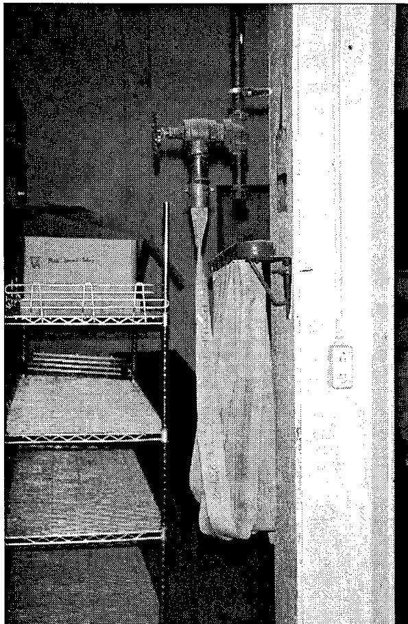
Figure 98. Fire hose located next to the collections storage area.
