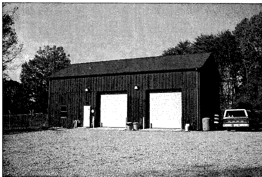
Figure 42. Exterior view of Storage Location 2, the maintenance building, at FLSHA.
