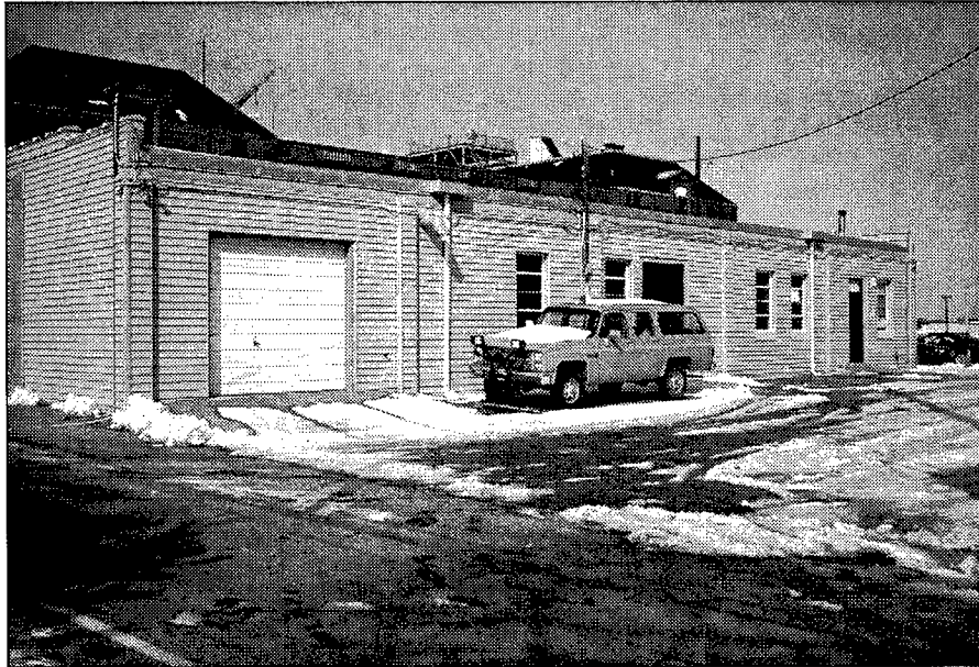
Figure 89. View of Storage Location 2, the storage facility used by USACE Baltimore District.
