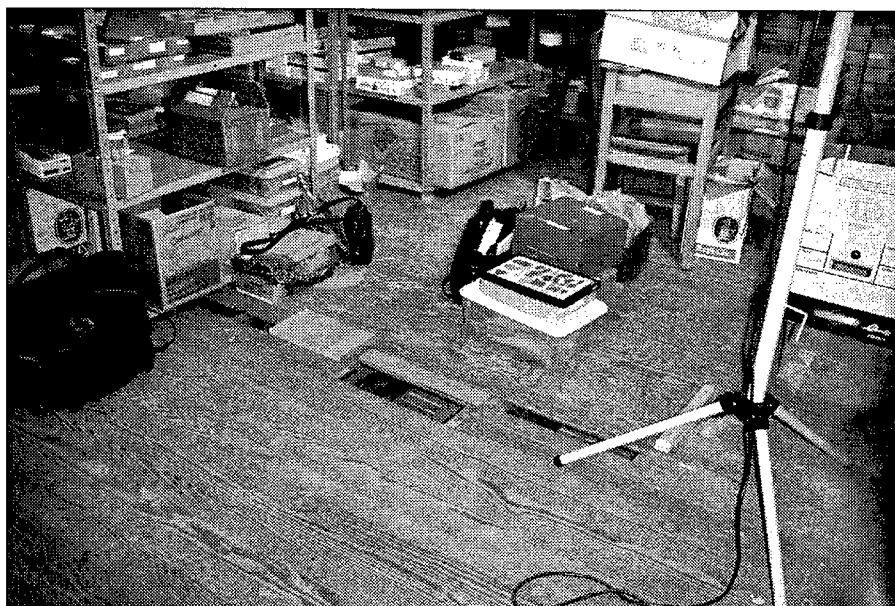
Figure 65. Missing floor boards are a safety hazard and the result of current repair work on the electrical system.
