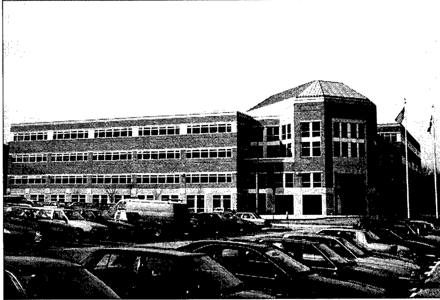
Figure 76. Exterior view of Storage Location 2, the PRC, at MHT.
