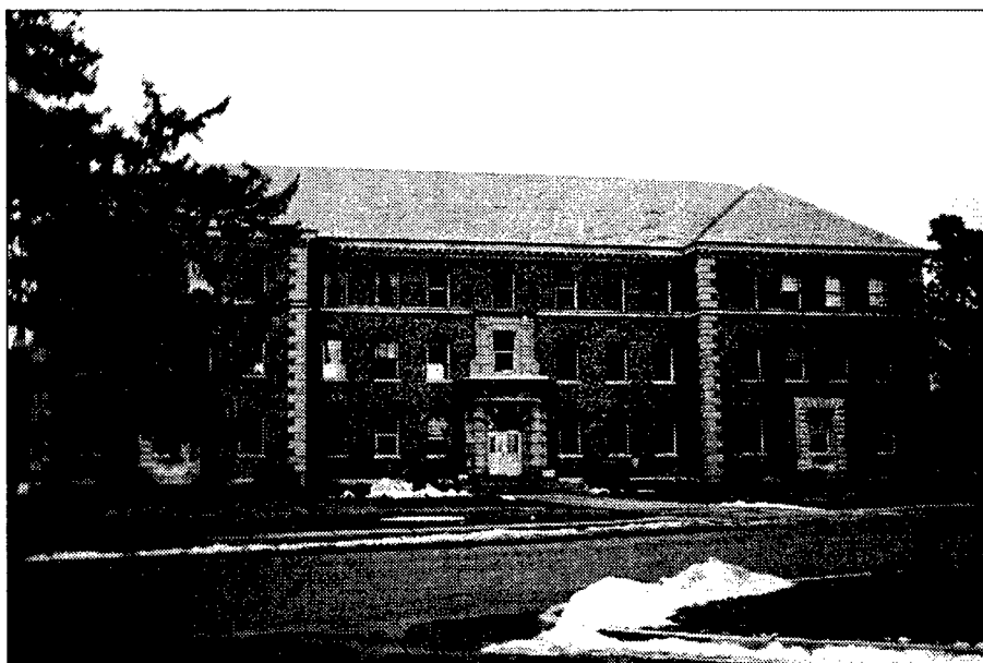
Figure 74. View of Storage Location 1, the Garrett building, at MHT.
