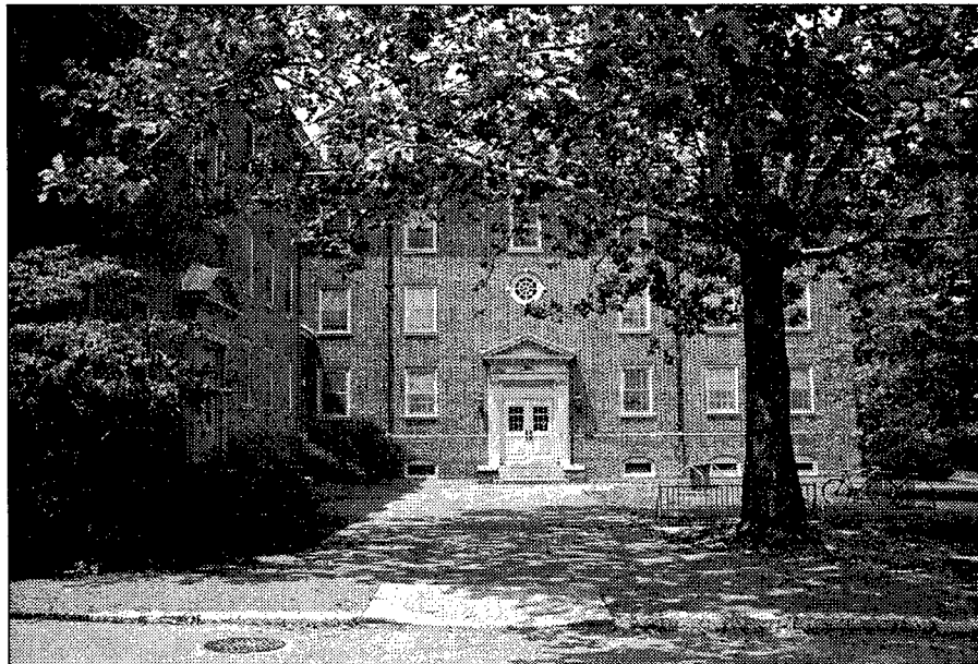
Figure 107. Exterior view of WMCAR. The basement of Camm Hall, a student dormitory, is used for collections storage.
