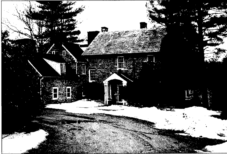
Figure 63. View of the Harford Glen Mansion. HCAS uses the attic as a collections storage area.
