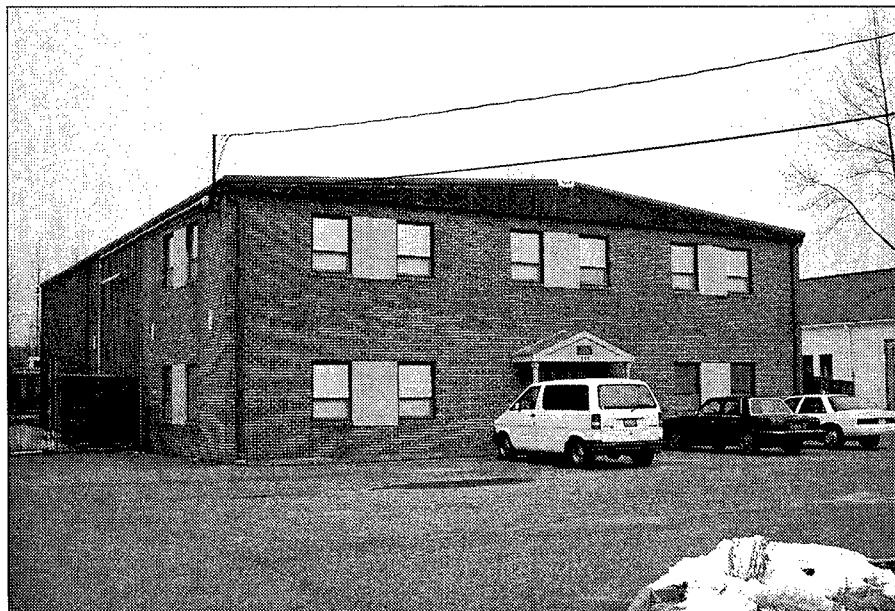
Figure 93. View of the building used by UDCAR.
