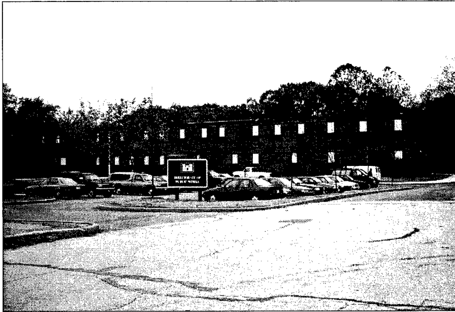
Figure 5. View of the DPW building that houses associated records and reports from Fort Belvoir.
