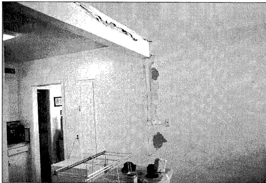
Figure 3. Water seepage through the roof damaged the paint on the interior rooms.
