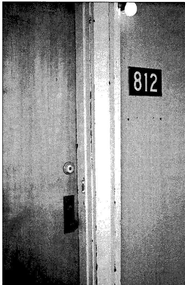
Figure 7. Key locks and double-cylinder, dead bolt locks are installed on both front doors to the Ellis Street lab.
