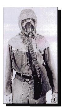
The need for a collective protection system for tank crews resulted in the development of the M14 Tank Mask in 1953. The facepiece was made of molded rubber in three sizes with a single plastic lens. A hose connected the mask to the air purifier and a cable connected a microphone to the tank's communication system. A standard canister was available when the mask was disconnected from the three-man collective protection system. A redesigned facepiece
