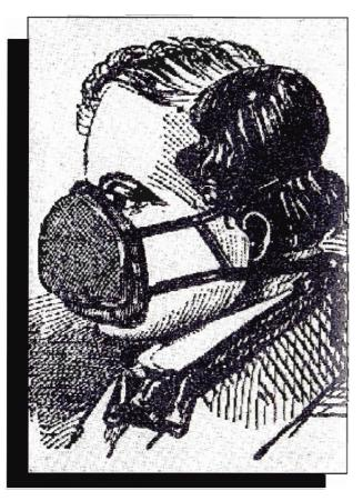
John Stenhouse, of Glasgow, Scotland, designed a mask in 1850 that used wood charcoal as a filtering material. The facepiece was velvet lined for a tight fit and used an elastic head band. Stenhouse did not patent his mask but gave it to the public. Within a few years, chemical manufacturers in London were supplying their workmen with charcoal respirators.
