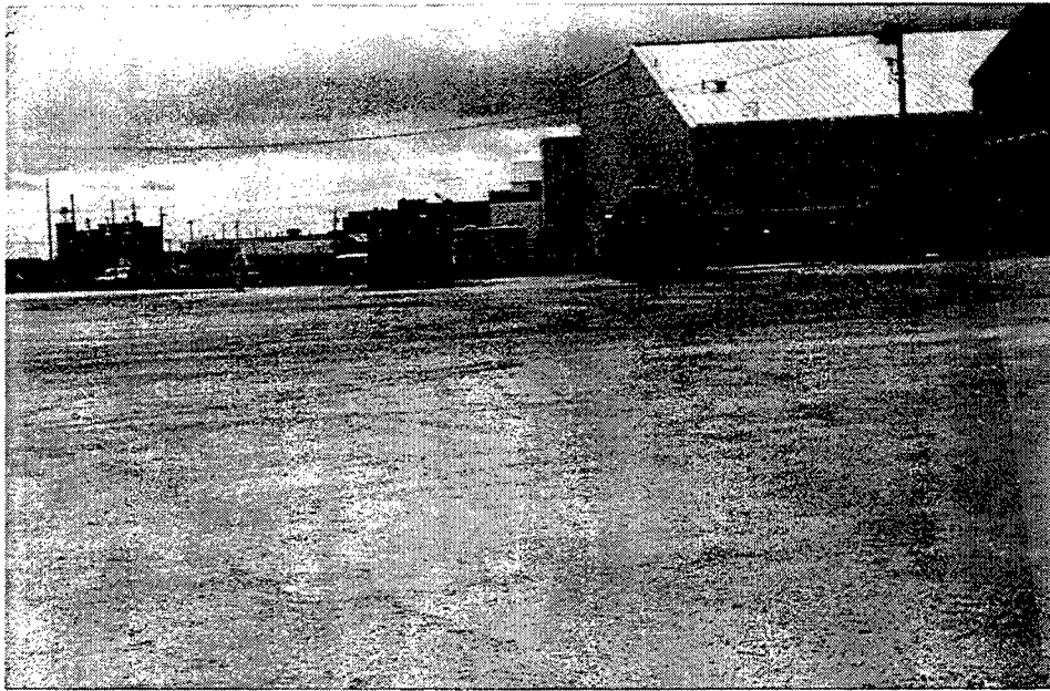
Figure 3.1: Overall view of RMP-surfaced fuel storage yard at Malmstrom AFB
