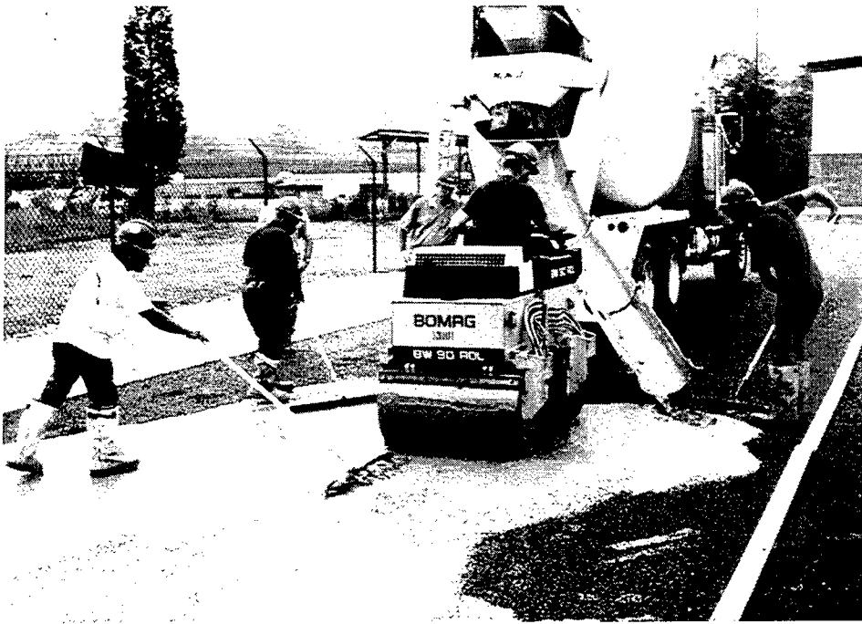
Figure 1.3: Typical view of applying grout to open-graded asphalt concrete surface
