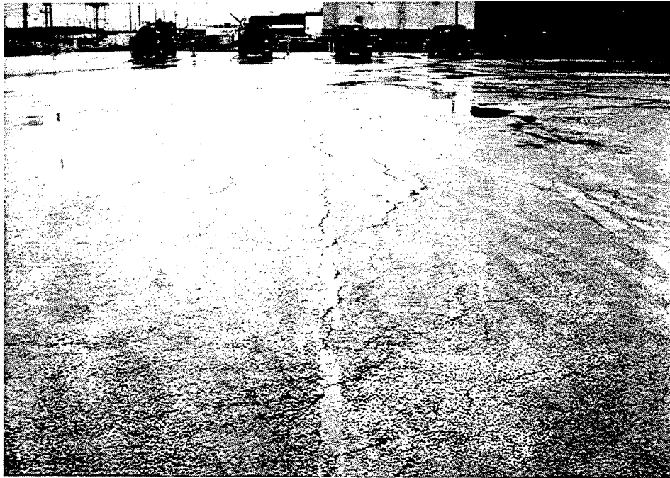
Figure 3.3: Isolated cracking and surface heaving in RMP caused by expansive clay subgrade at Malmstrom AFB
