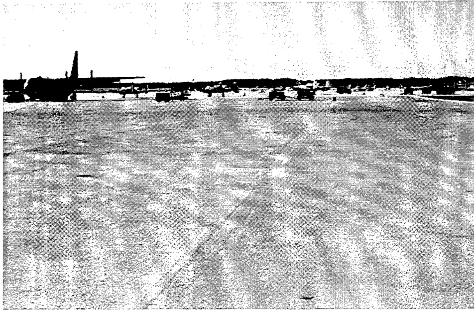
Figure 3.11: Overall view of RMP-surfaced Hanger 6 Apron
