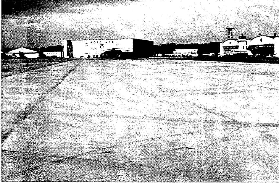
Figure 3.8: Overall view of RMP-surfaced Snack Bar Apron
