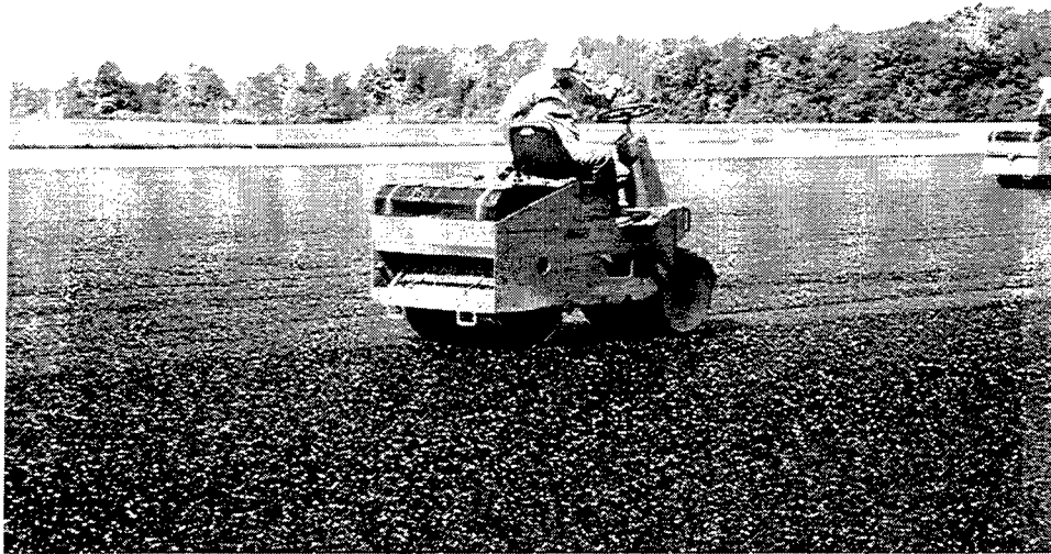
Figure 1.2: Typical view of rolling open-graded asphalt concrete with steel-wheel roller
