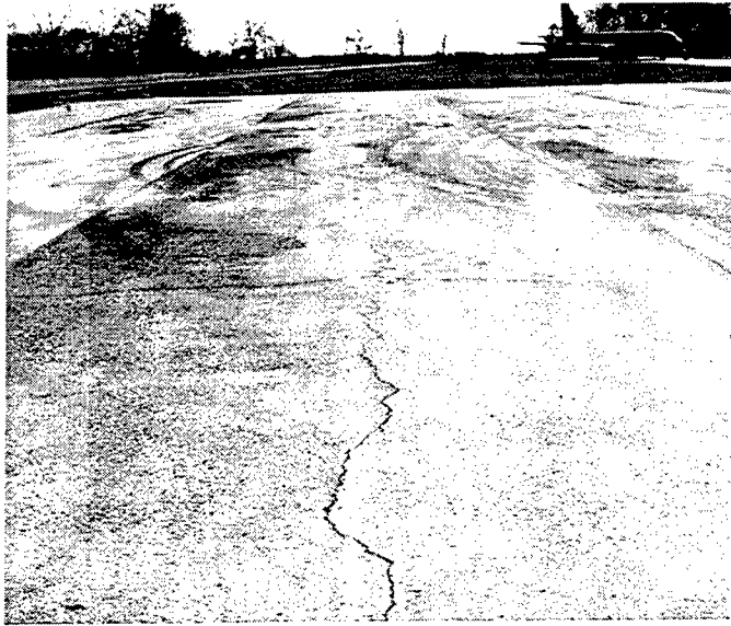
Figure 3.14: Reflective cracks in RMP apron at Fort Campbell Army Airfield
