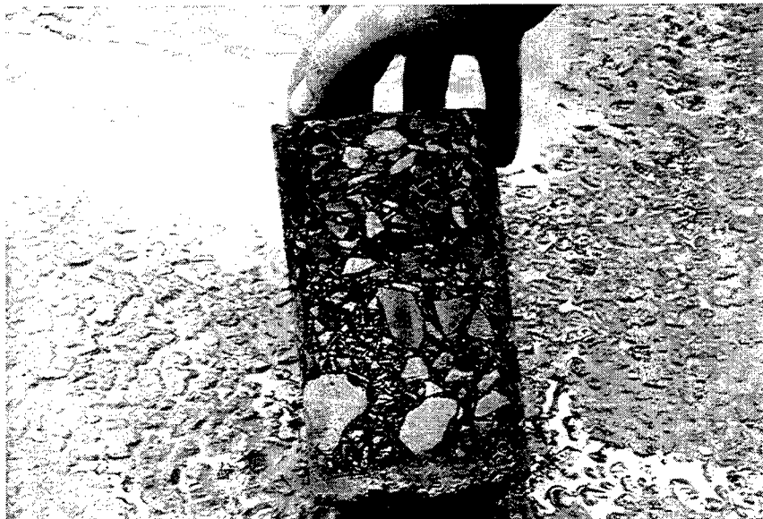
Figure 3.16: Core sample from RMP at Altus AFB showing complete penetration of grout into open-graded asphalt layer
