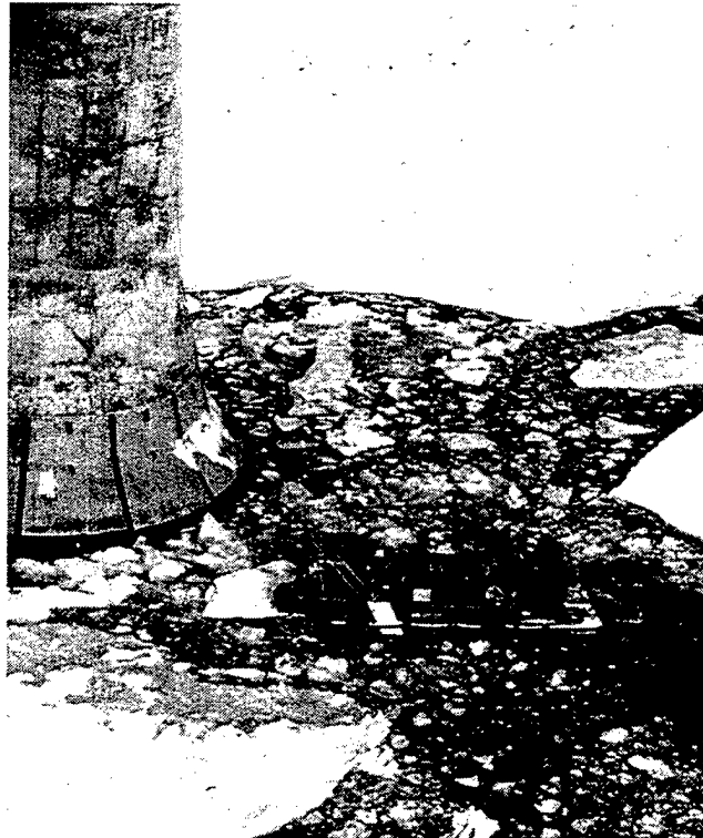
Figure 2 Ice Forming around the Bridge Pier
