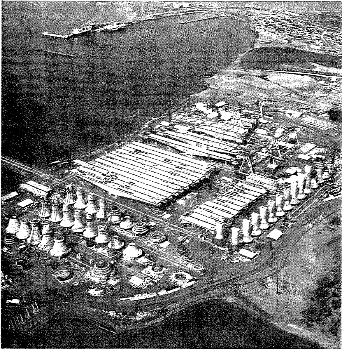
Figure 6 The Precast Yard Layout and Various Stages of Production of the Pier Bases and the Main Girders
