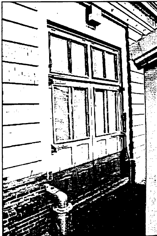
Figure 66. Drainage Pumping Station No. 7. Wooden vehicle door on west end of building.
