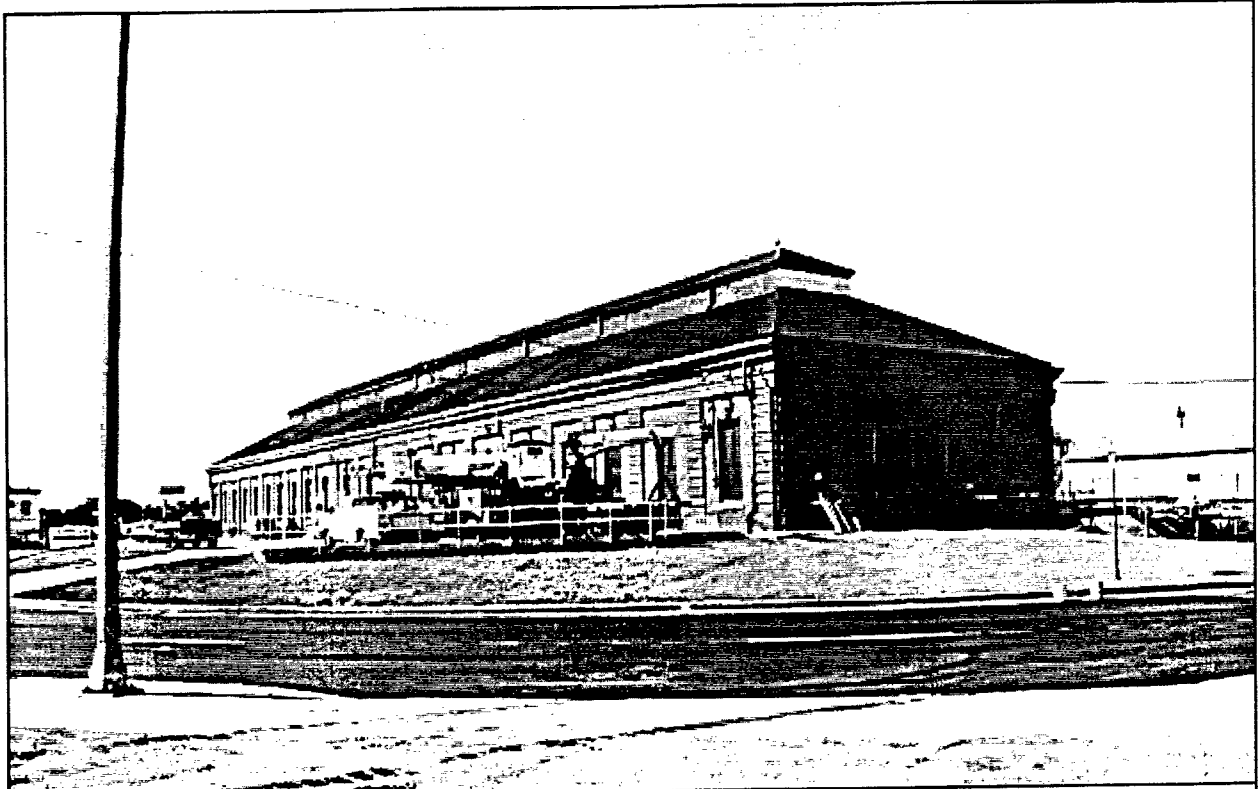
Figure 30. Drainage Pumping Station No. 1. View looking southwest.
