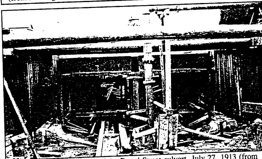
Figure 75. Interior view of the Broad Street culvert, July 27, 1913 (from Louisiana Collection, Howard-Tilton Memorial Library, Tulane University).
