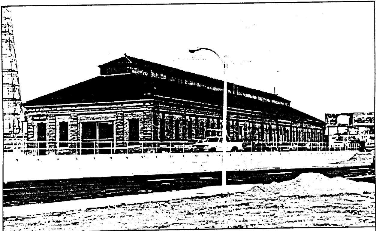
Figure 31. Drainage Pumping Station No. 1. View looking northwest.
