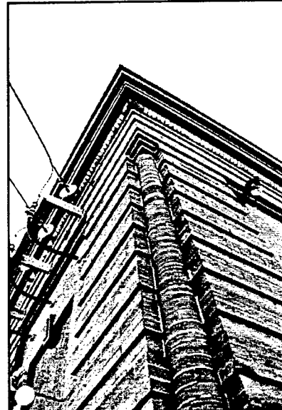
Figure 85. Drainage Pumping Station No. 1. View of upper portion of east facade of building, showing pilasters, wall, and entablature, quarter-round bricks at transition to cornice, and decorative cast-metal false key-stone on window.
