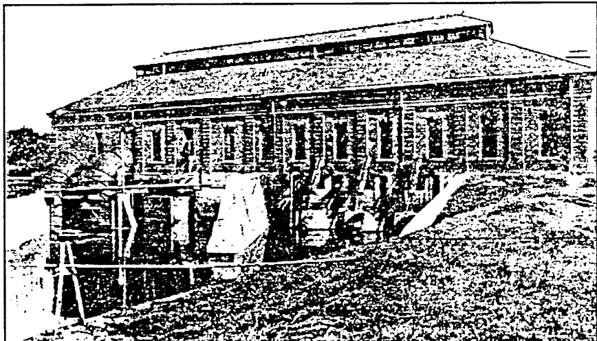
Figure 23. Exterior of Drainage Pumping Station No. 1, after alteration for 12' Wood screw pumps, photographed ca. 1915-1926 (from Sewerage & Water Board n.d.).
