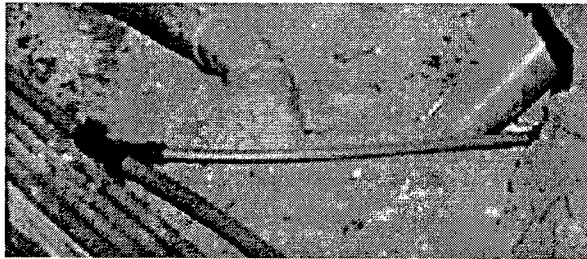
Fig 5: Y-branch as applied in connecting the MCJ with the customer premise
