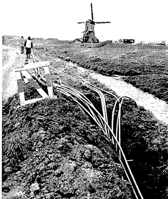
Figure 1 Laying of HDPE protective tubes in the Netherlands for the optical backbone-network.
