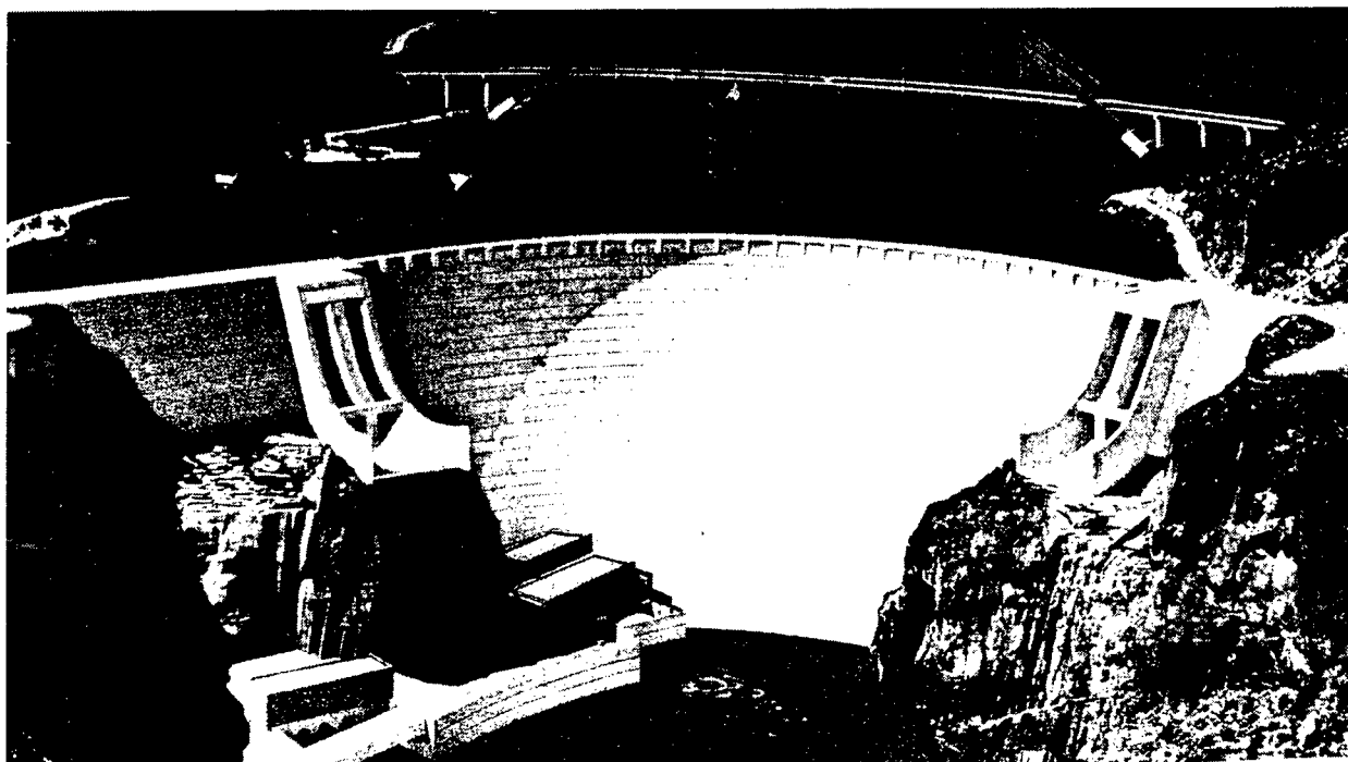
Figure 105. Modifications performed at Theodore Roosevelt Dam
