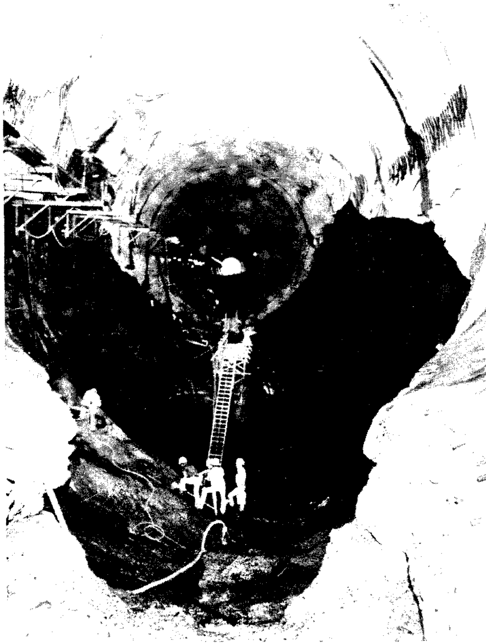
Figure 93. Cavitation damage downstream of the elbow in the left spillway elbow at Glen Canyon (from Burgi and Eckley 1987)
