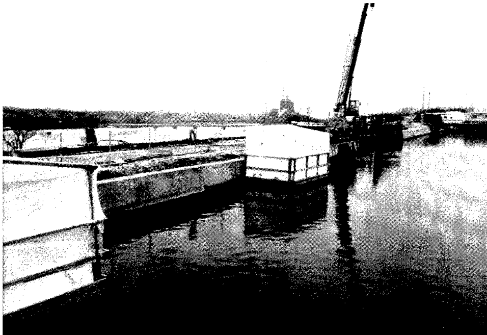
Figure 15. Head gate section on upstream face at Brandon Road Dam after rehabilitation
