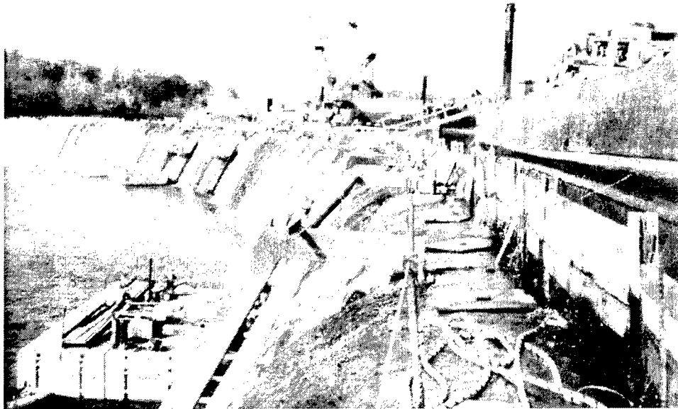
Figure 121. Typical spillway repair in progress at Crescent Dams (from Sumner, Nash, and Haag 1991)
