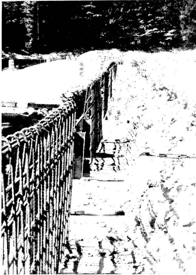
Figure 56. Construction of a parapet wall on the upstream crest of Mohawk Dam (from U.S. Army Engineer District, Huntington 1990b)
