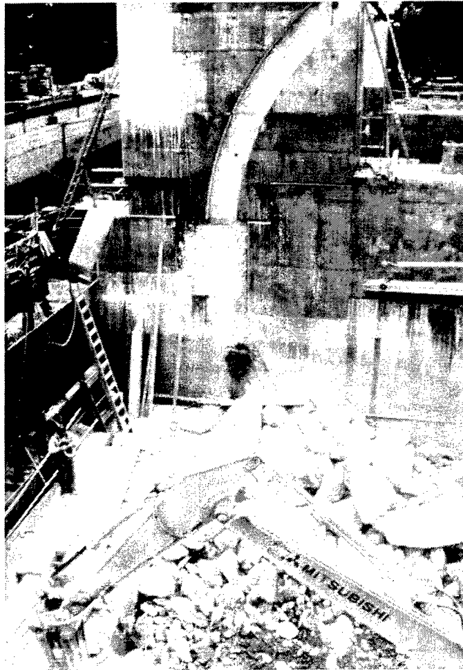
Figure 29. Concrete removal of ogee crest and side of pier to accommodate new gate, Marseilles Dam
