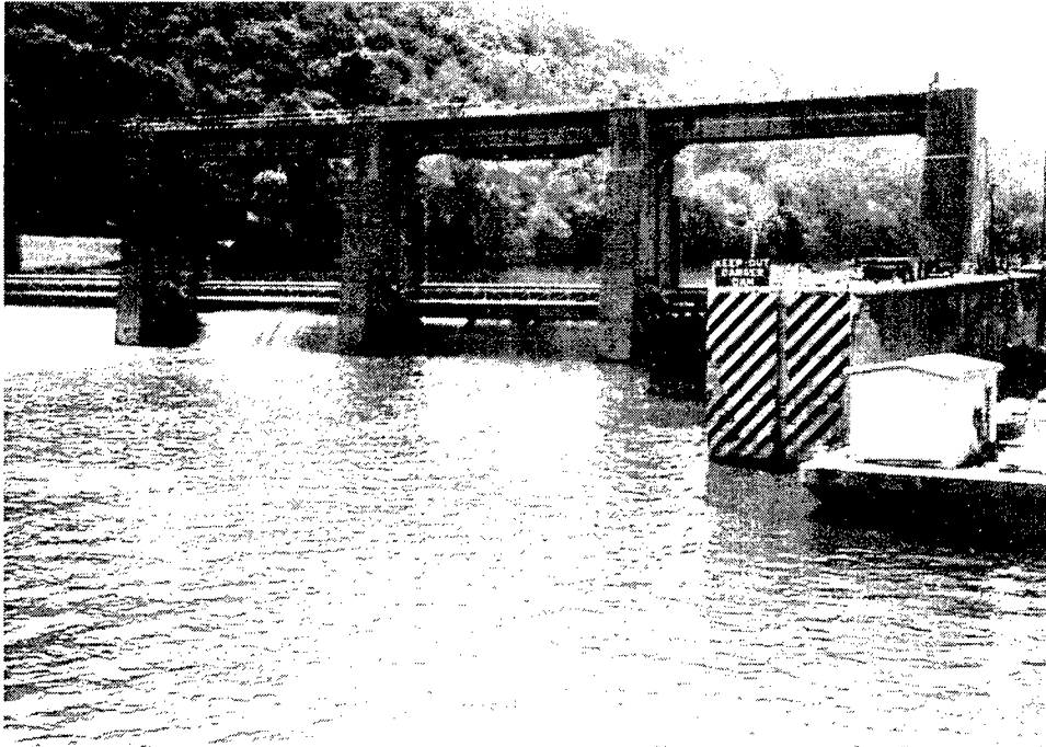
Figure 72. Downstream face of Point Marion Dam; end of old land wall is at right (from U.S. Army Engineer District, Pittsburgh 1994)
