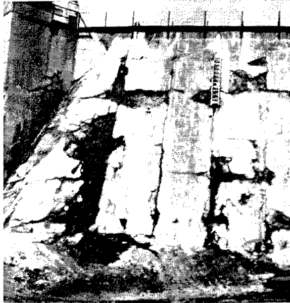
Figure 114. Deteriorated shotcrete repair on the downstream face of Big Eddy Dam (from Gore and Bickley 1987)
