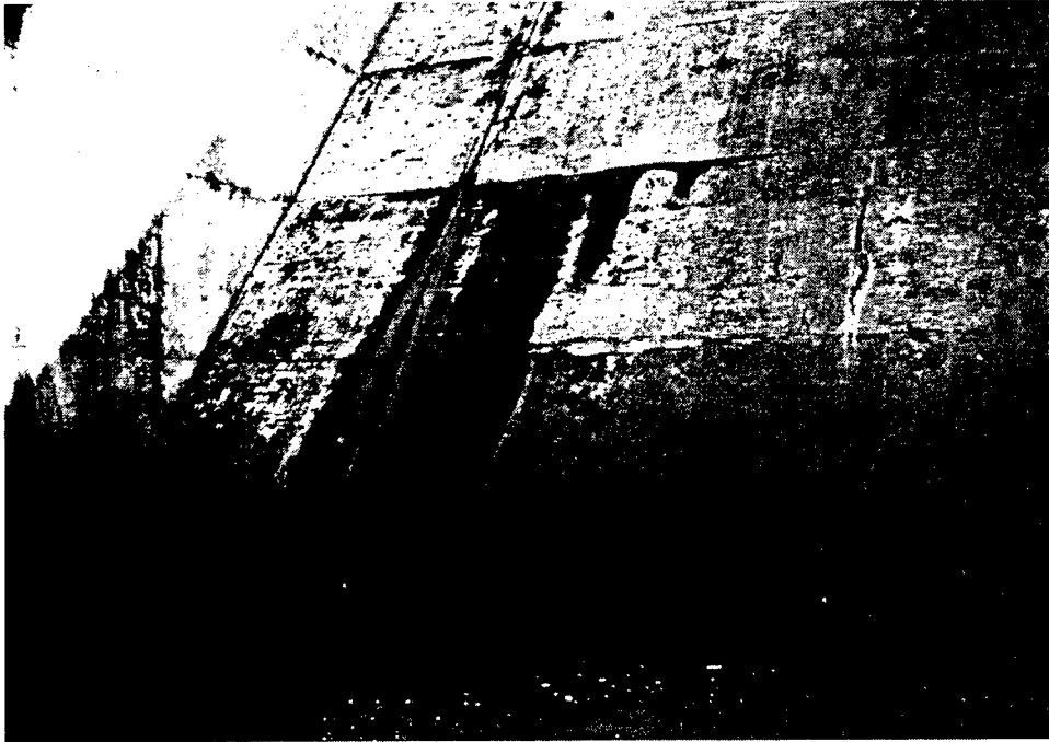
Figure 78. Leakage at monolith joint 5/6, Stonewall Jackson Dam (from U.S. Army Engineer District, Pittsburgh 1989b)
