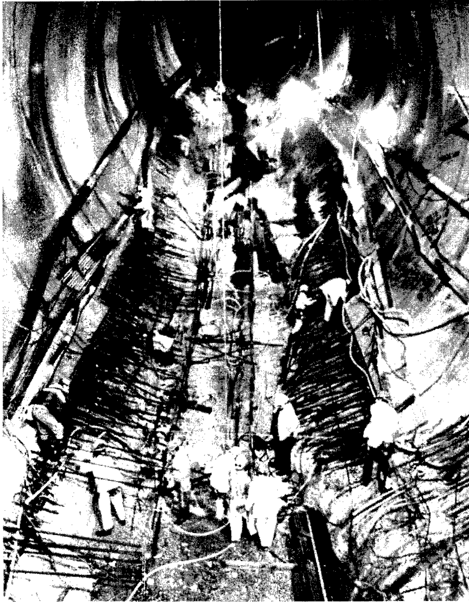
Figure 94. Steel reinforcing steel being replaced in the invert of the spillway elbow at Glen Canyon (from Burgi and Eckley 1987)
