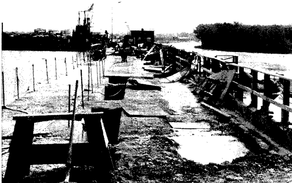
Figure 16. Repairs to the horizontal deck of the head gate section at Brandon Road Dam
