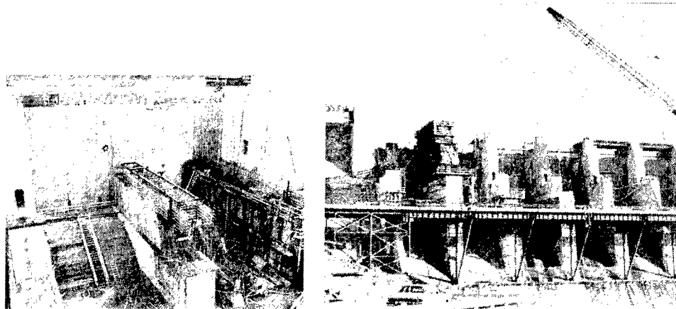
Figure 44. Piers raised and widened to resist greater head at Chief Joseph Dam (from ENR 1978)
