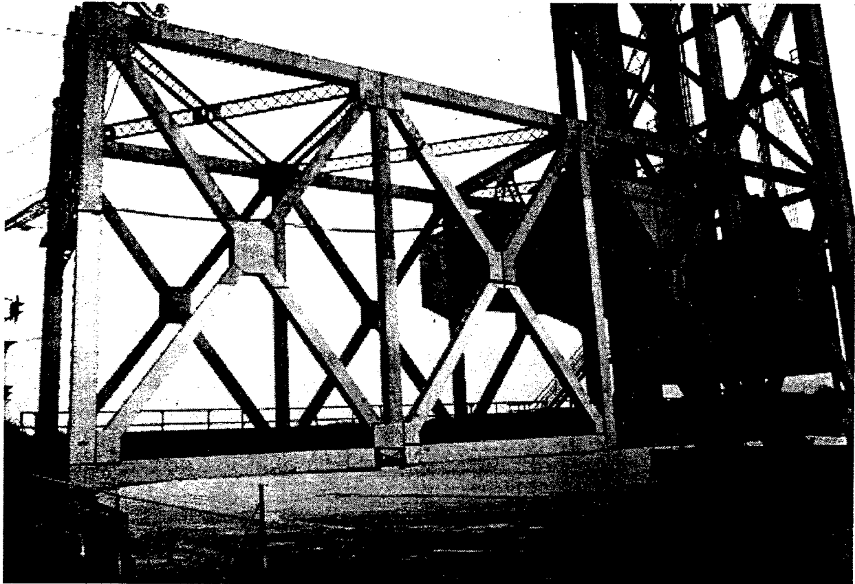
Figure 2. Segment of railroad bridge over Cape Cod Canal used for 1994 coatings field test.
