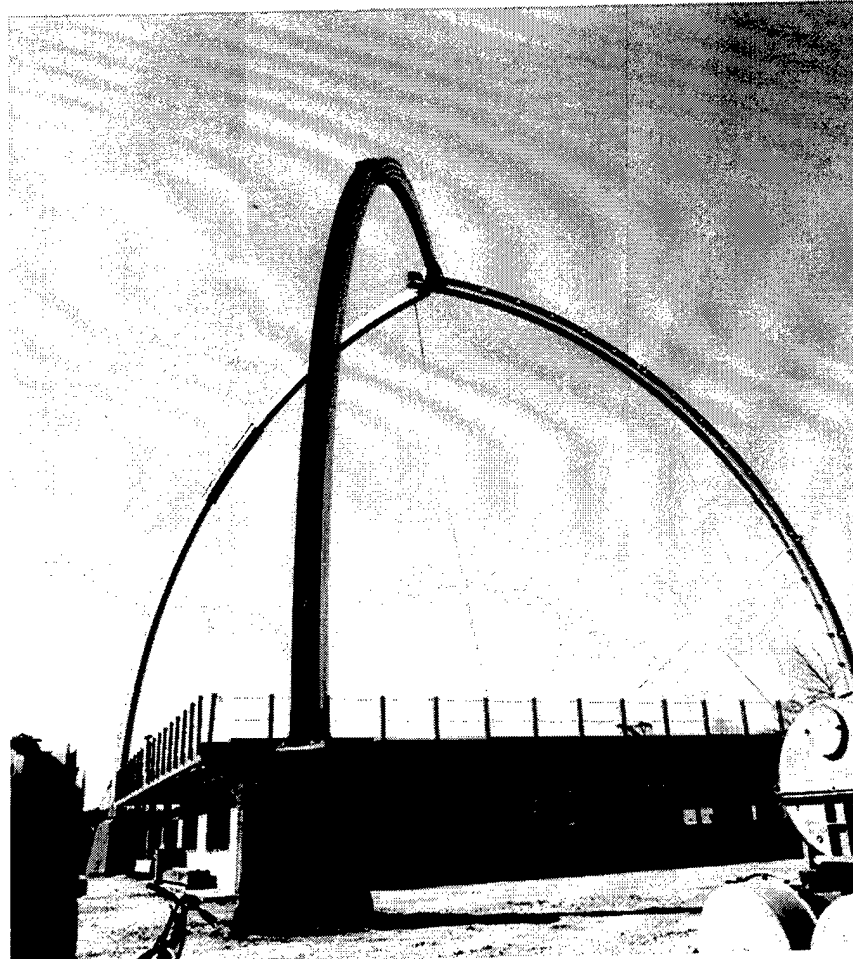
Overwater Antenna Test Range Facility, New London
