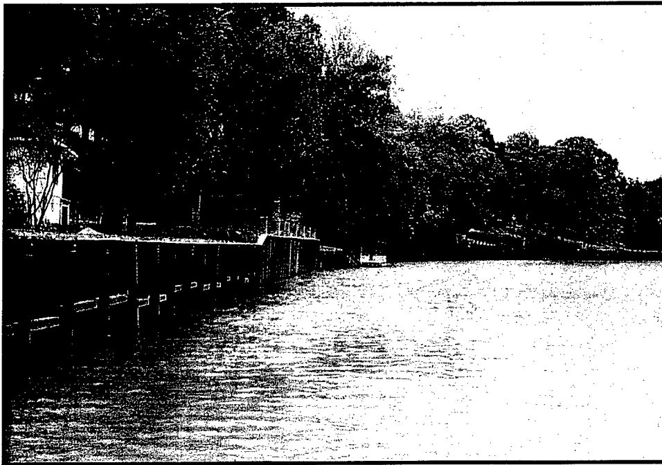
Figure 23. Composite bulkheads fabricated from steel and wood that line the riverbank along much of the Vermilion River survey area were a frequent source of the large magnetic disturbances recorded during the survey.
