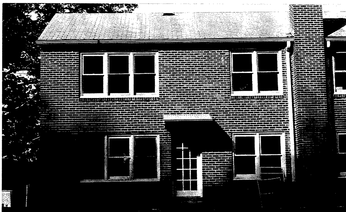
Figure B-12. House 1330H, Rear View
