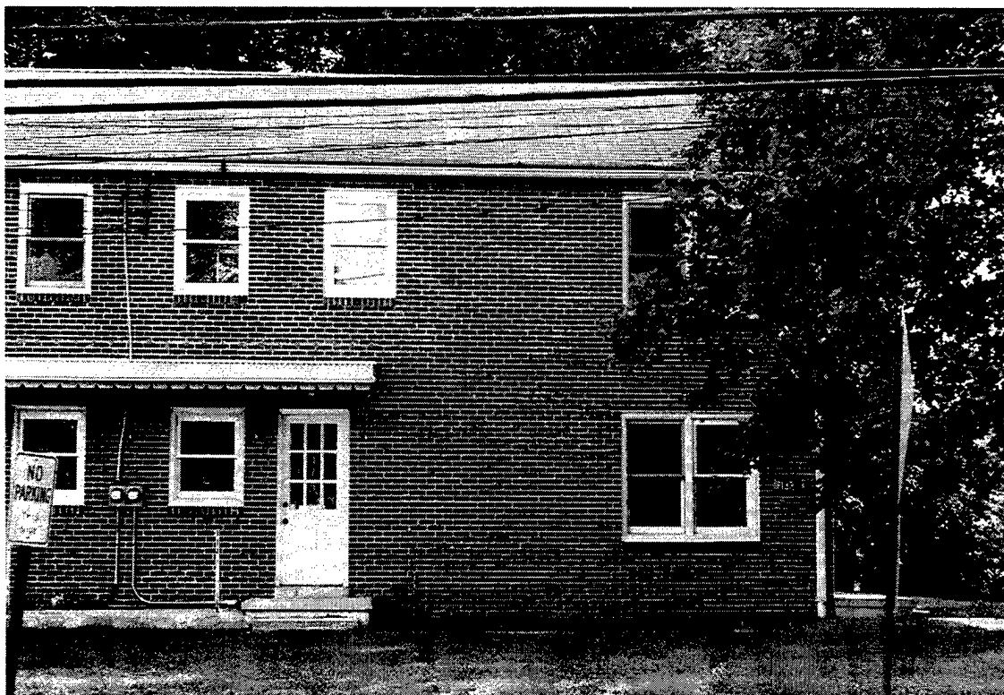
Figure B-11. House 1330H, Front View
