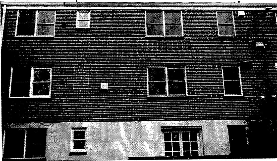
Figure B-14. House 1342A, Back View
