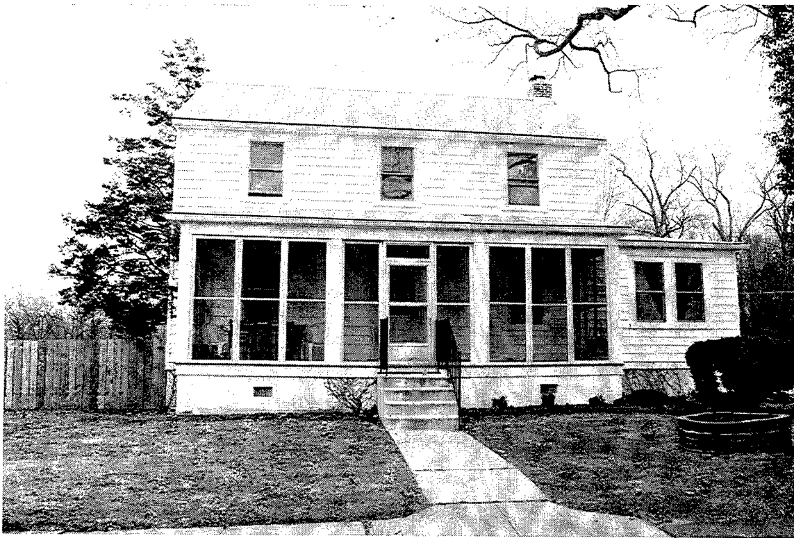
Figure B-8. House 1236, Back View
