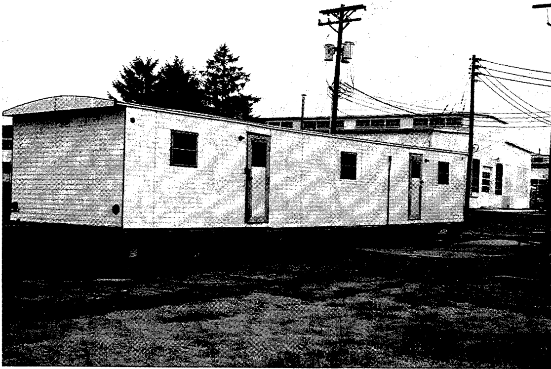
Figure B-23. Trailer 5354, Front View
