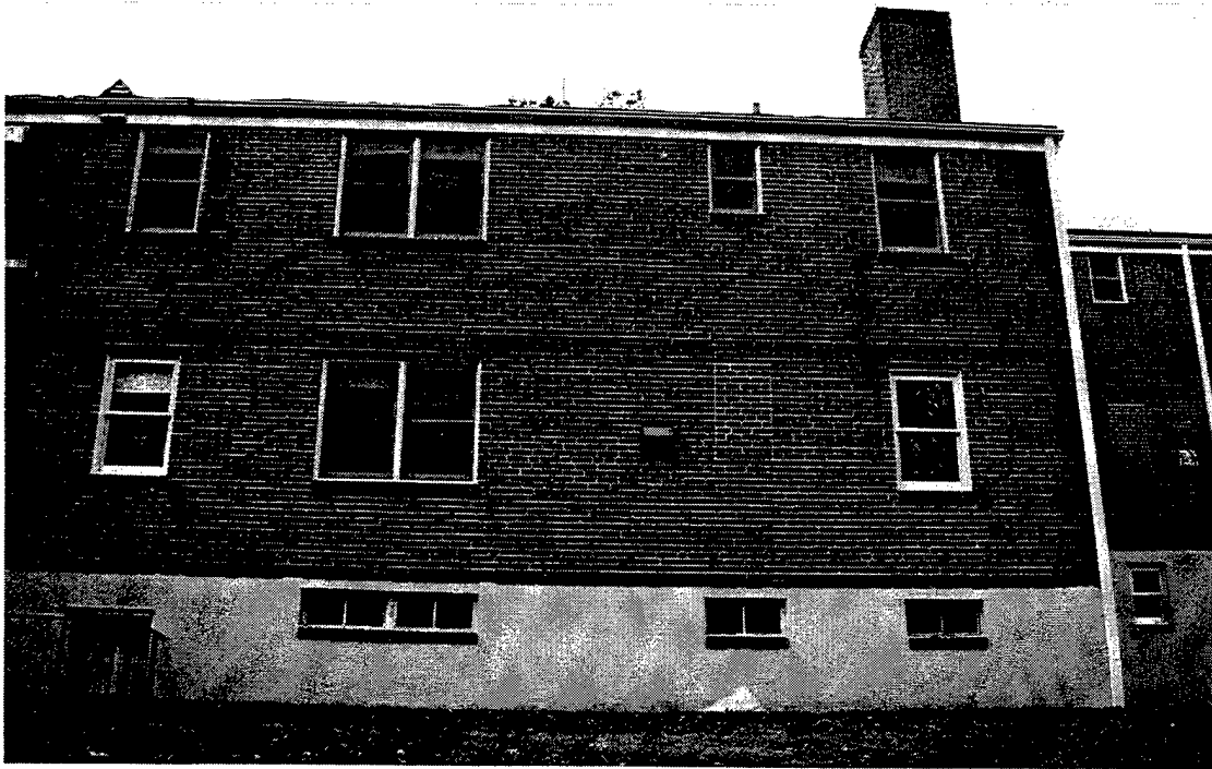
Figure B-16. House 1345B, Rear View
