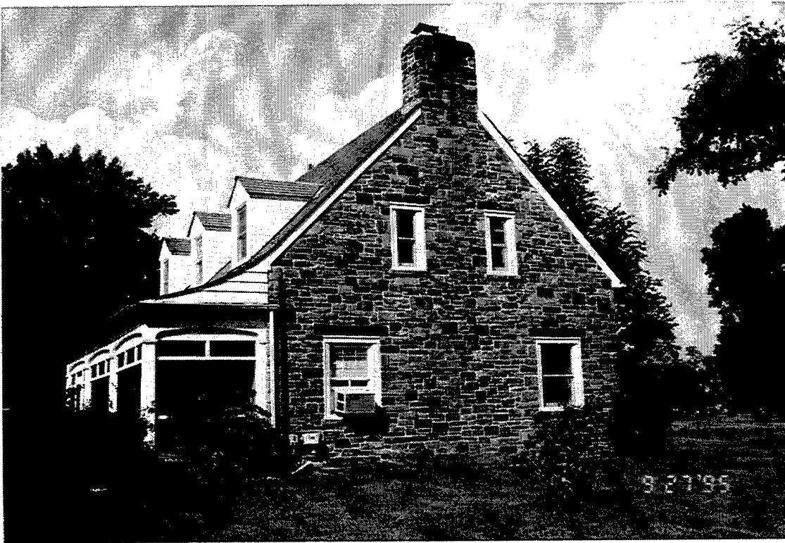
Figure B-2. House 54, Side View
