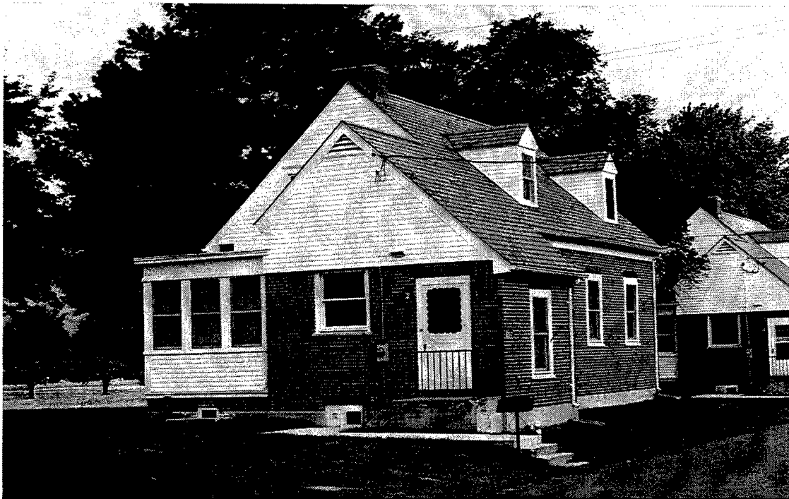
Figure B-20. House 3069, Side View
