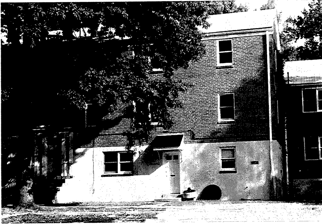
Figure B-13. House 1342A, Front View
