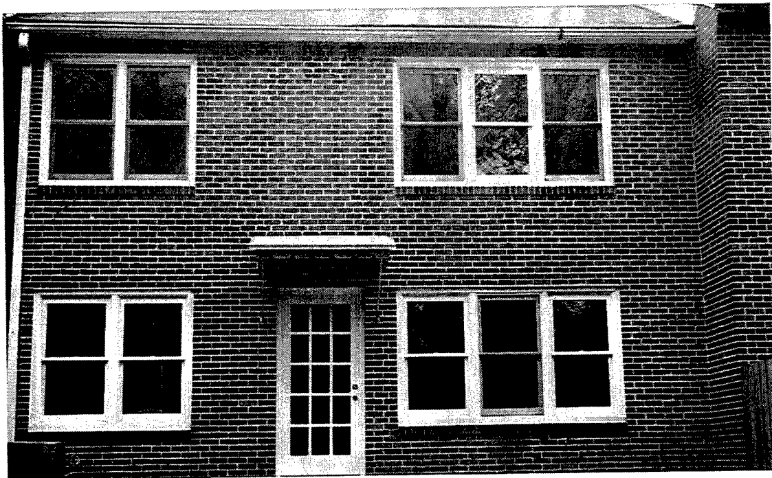
Figure B-10. House 1330G, Back View
