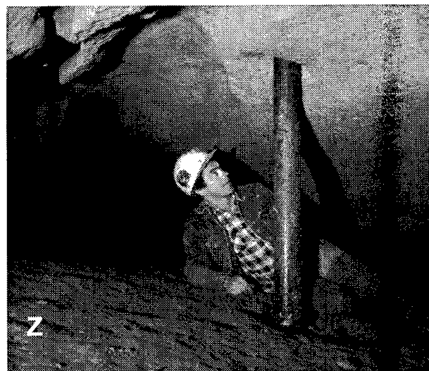
Typical karst problems (see also Photo B): Y : Because of rapid transit times and lack of filtering, water in karst conduits is usually of low quality and subject to severe contamination (Onesquethaw Cave, N.Y.). Z : If water wells encounter active conduits, they should be cased and sealed (Blue Spring Cave, Ind.). ZZ : Artificial drain in sinkhole, Bowling Green, Kentucky, installed to prevent depression from filling with water during heavy rains. Subsidence of overburden in the sinkhole floor has damaged the drain.
