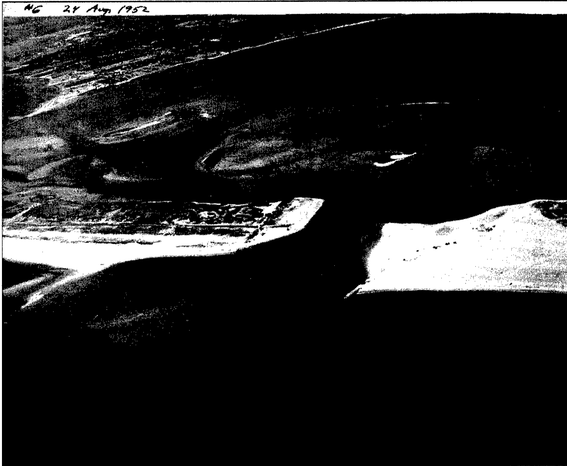
Figure 10. Photograph taken during construction of east jetty, 24 August 1952 (Channel runs northeast-southwest, closely following revetment on west shoreline and heads out to sea just east of a spit on Tiana Beach. Ebb shoal has an almost straight seaward margin. On flood shoal, three channels merge at bay end of inlet. Two of these channels, east and central, have shoaled) (Westhampton Photo Studio, from Suffolk County Department of Public Works)
