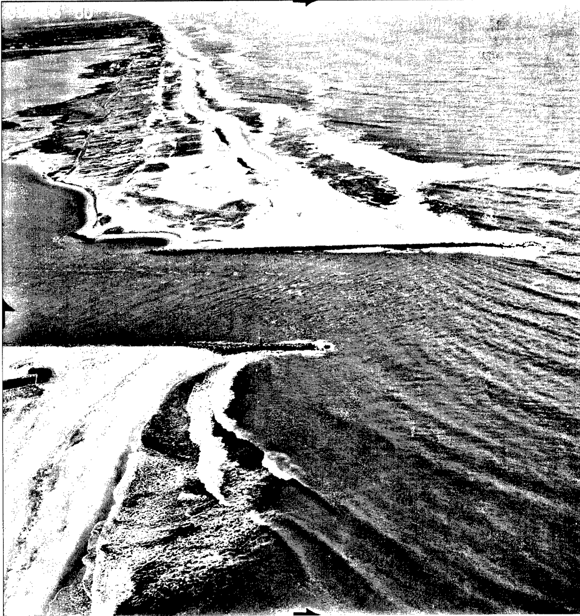
Figure 13. View east, with Atlantic Ocean to right, 18 January 1980 (Triangular-shaped updrift fillet is pronounced just beyond east jetty. Original, pre-inlet dune line approximately followed white line that marks dune crest in distance. Road paralleled dune crest and continued west before inlet was cut in 1938. Tip of west jetty has deteriorated. Remains of 1940 revetment are not visible in this image) (Topo-Metrics image 08013 0-16)
