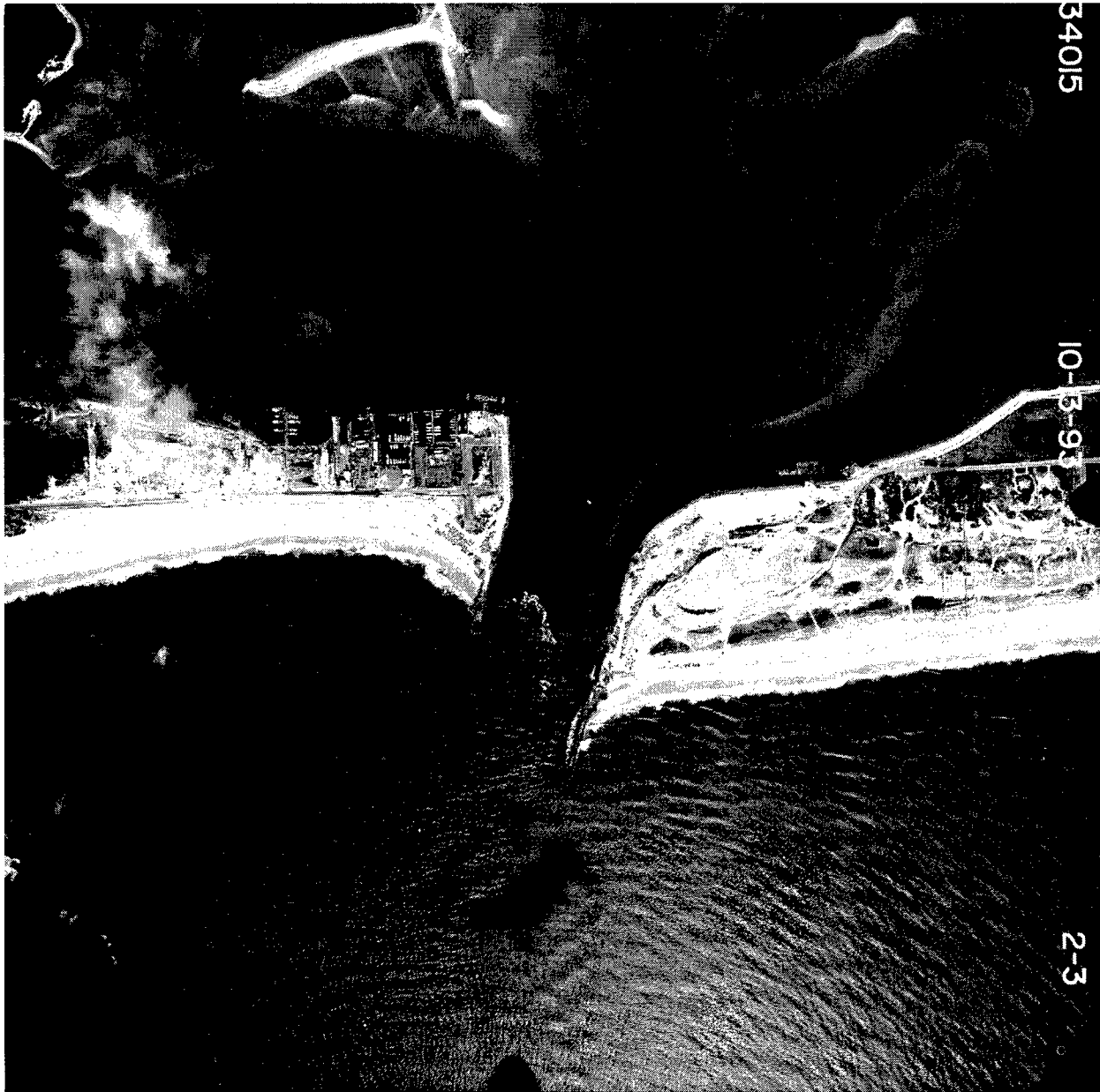
Figure A42. 13 October 1993 (Ocean shorelines have not changed since the previous photograph was taken in June. Repair of the east revetment is almost complete)
