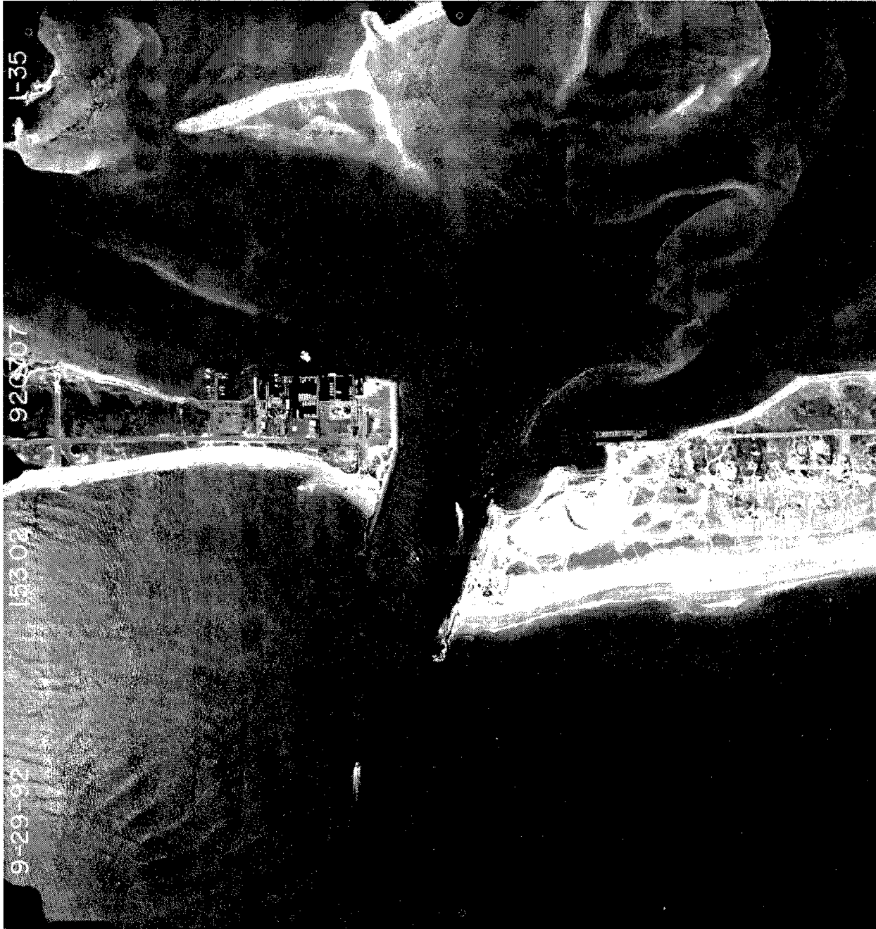
Figure A36. 29 September 1992 (East beach has advanced about 70 m compared with December 1991, and west beach has receded severely. More of the east revetment has deteriorated, accompanied with erosion of east shore. Jetty repair has begun, and a barge containing rock is moored in east channel in Shinnecock Bay. On the flood shoal, the right arm of the T-shaped sandbar has moved north)
