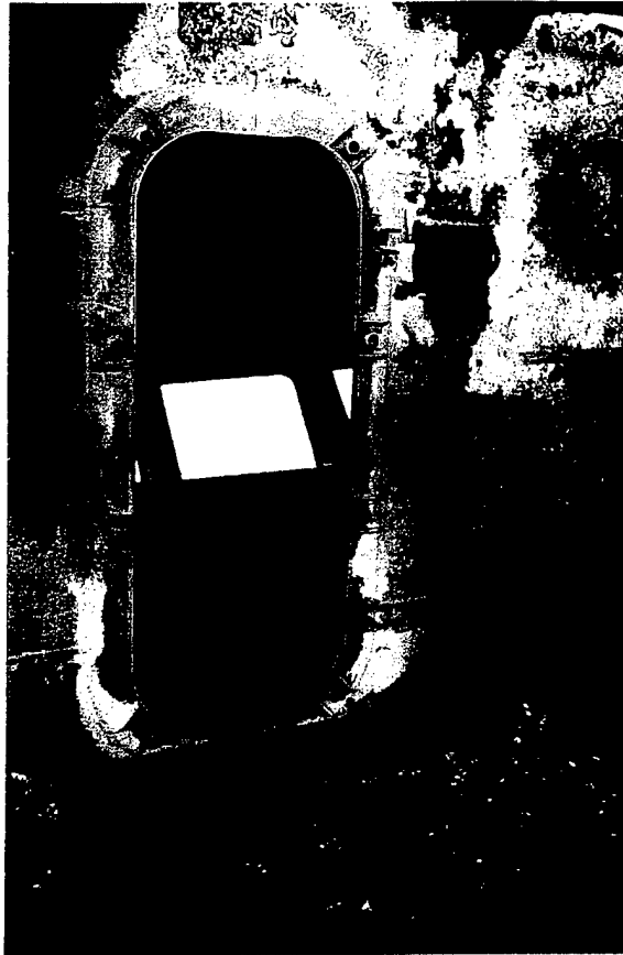
Fig. 8 — Vent opening in Berthing 2 hull structure, viewed from well deck
