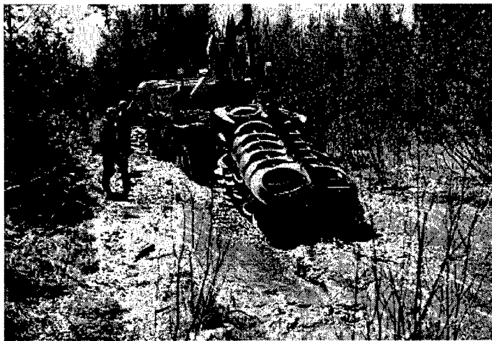
Figure 5. Placing tire mats onto wooded trail section.
