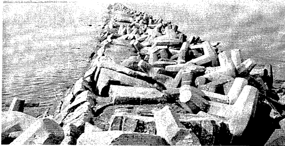
Figure 43. View of 1,814-kg (2-ton) dolosse along trunk of Cleveland Harbor east breakwater
