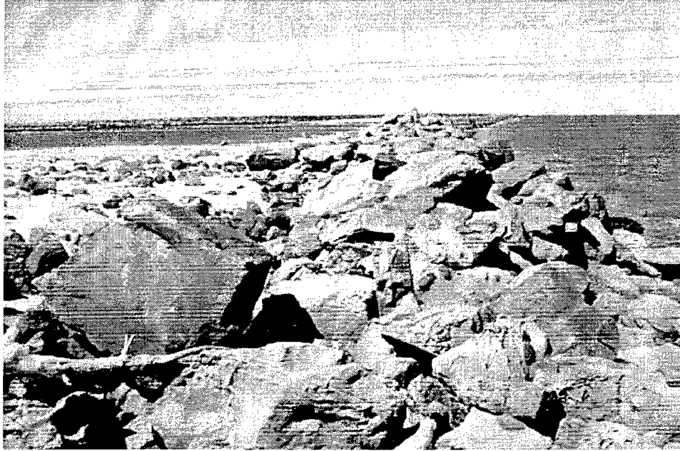
Figure 23. Scattered armor stone on shore side of Umpqua training jetty
