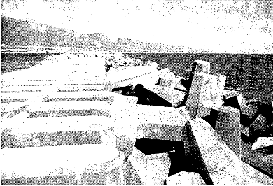
Figure 6. Kahului east breakwater
