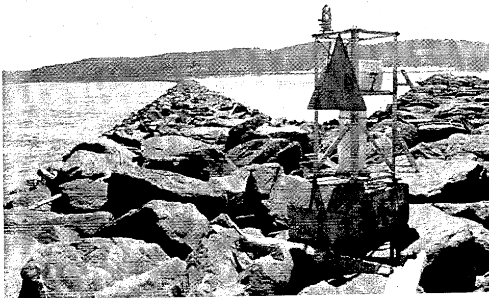
Figure 22. View of Umpqua River training jetty (left structure) looking shoreward
