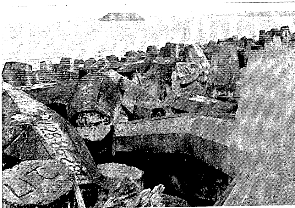
Figure 28. View of 38,100-kg (42-ton) dolosse on the sea-side slope of the main stem of the Crescent City breakwater
