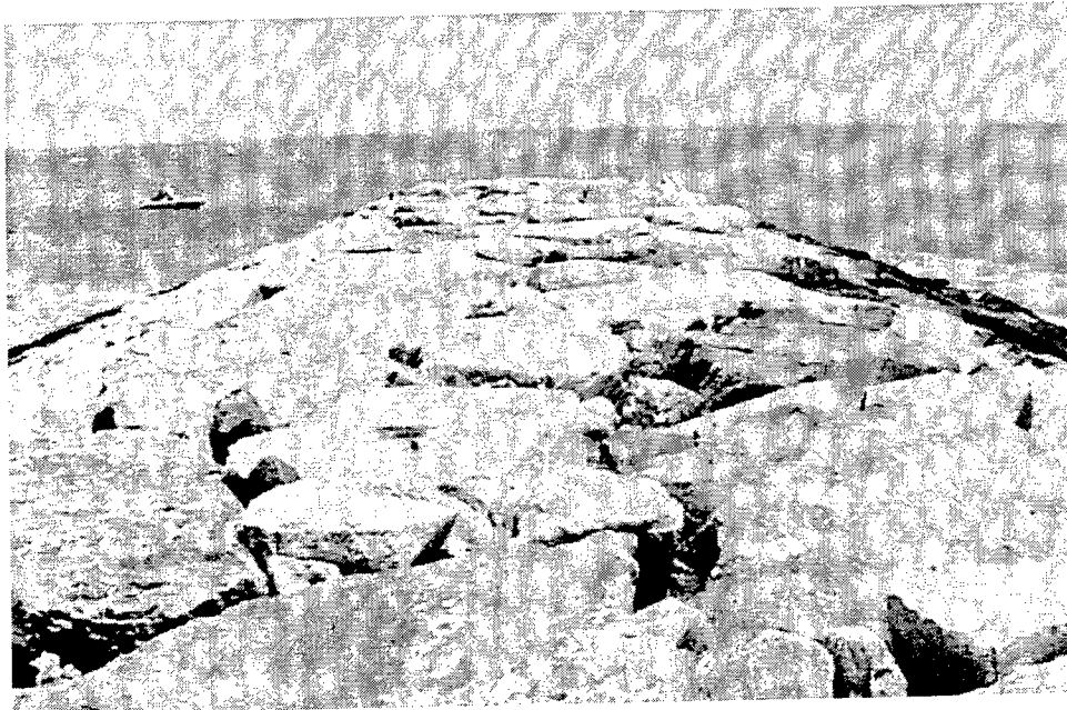
Figure 55. Head portion of south jetty rehabilitation at Ocean City Inlet
