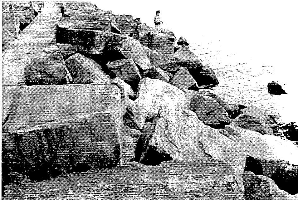
Figure 46. Void along trunk (sta 16+50) of Cattaraugus Creek south breakwater
