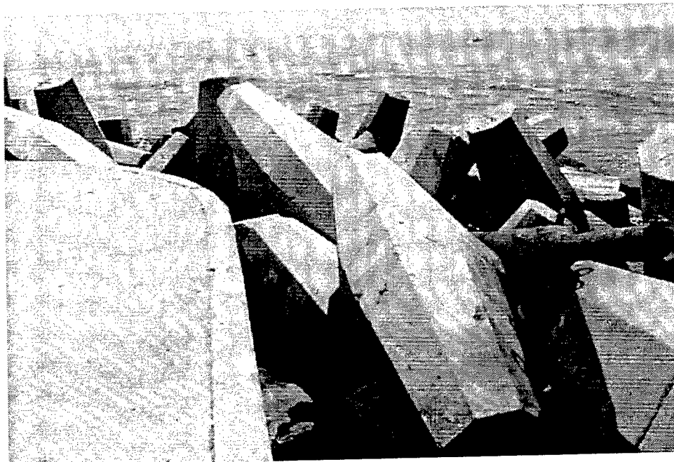
Figure 49. 14,515-kg (16-ton) dolos armor units on Manasquan Inlet jetties
