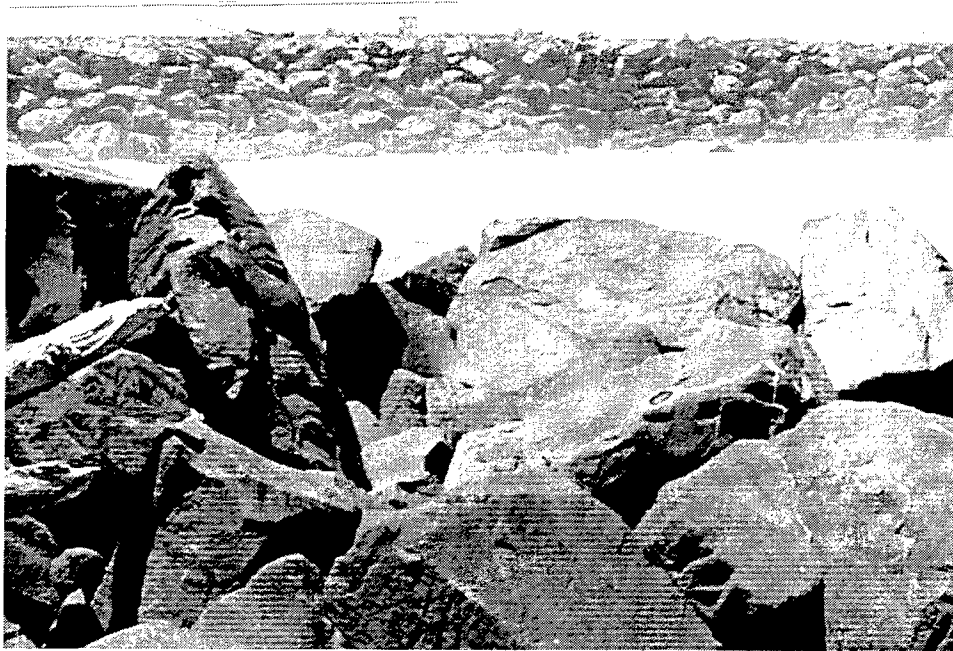
Figure 17. Displaced stone on north jetty spur at Siuslaw
