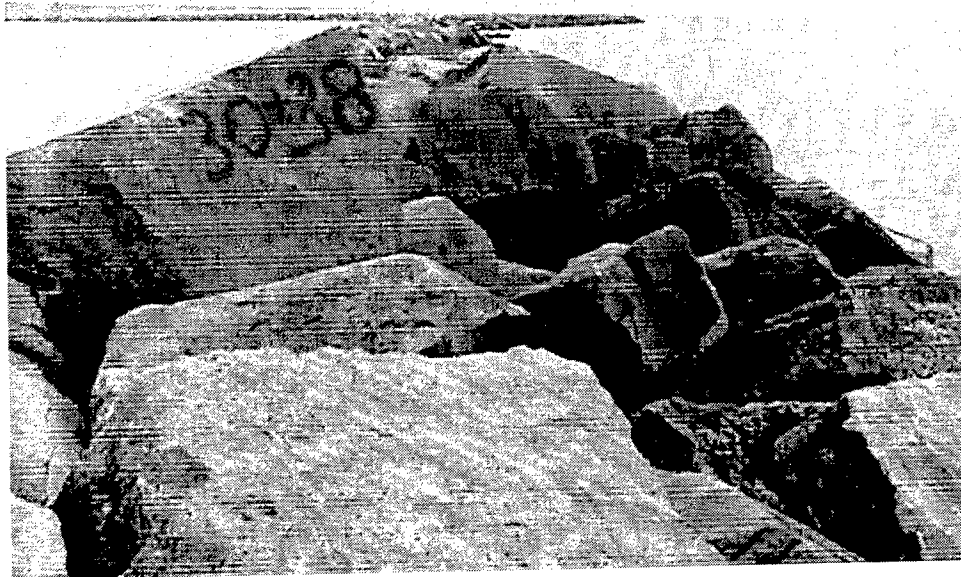
Figure 38. Burns Harbor breakwater looking west
