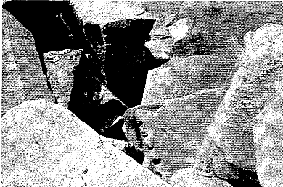
Figure 39. Void on lakeward crest of Burns Harbor breakwater
