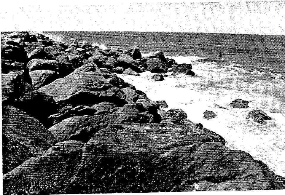
Figure 13. Head of Yaquina Bay north jetty on 24 June 1997
