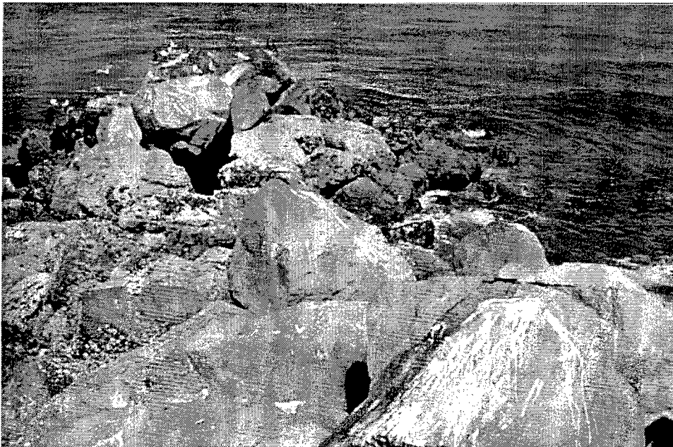
Figure 24. Breach at head of Umpqua River south jetty
