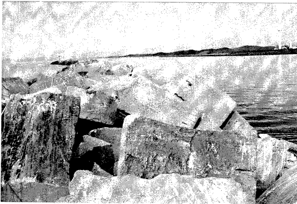
Figure 37. Burns Harbor breakwater looking east
