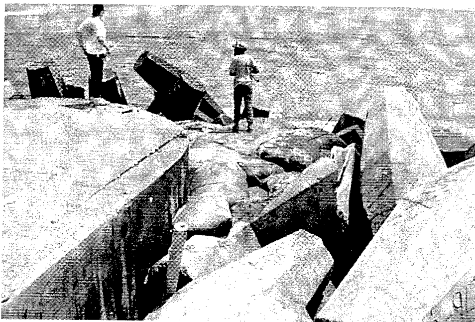
Figure 51. Emergency repair work (grout-filled bags) at head of Manasquan Inlet south jetty
