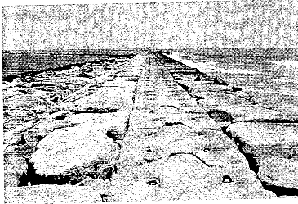
Figure 54. Rehabilitated south jetty trunk at Ocean City Inlet
