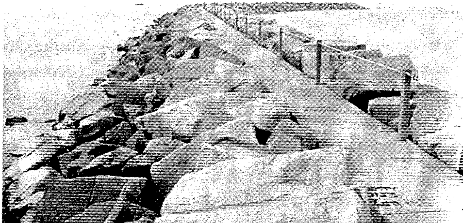
Figure 45. Cattaraugus Creek south breakwater looking lakeward
