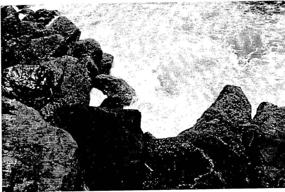
Figure 20. Void in south jetty spur at Siuslaw
