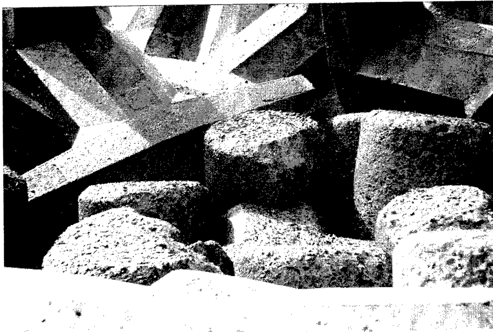
Figure 4. Surface spalling of tribars on Nawiliwili breakwater
