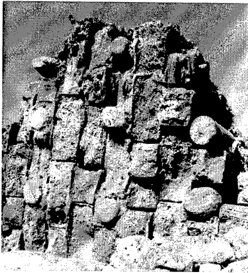
Figure 56. Section of Citadel Tower. (View east). One of a few large remaining sections of the tower and wall. Ashlar and mortar construction tied together with granite columns.
