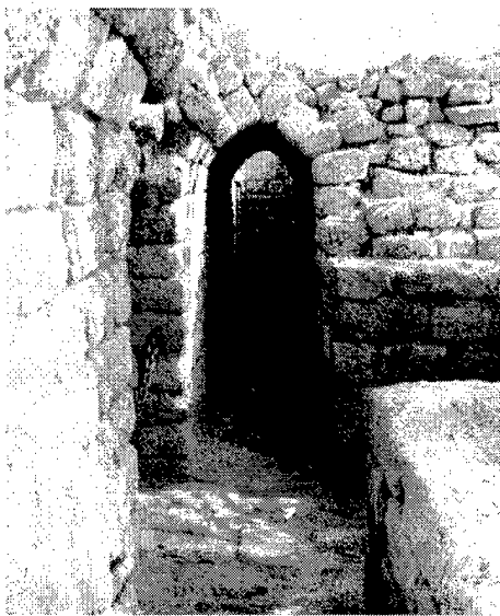
Figure 43. East Gatehouse Upper Balcony. (View north, east wall inside access hallway). On the left, balcony opens into vaulted ceiling of gatehouse. On the right, archer's loophole. At the end of the hallway, stairway up to the projecting tower.
