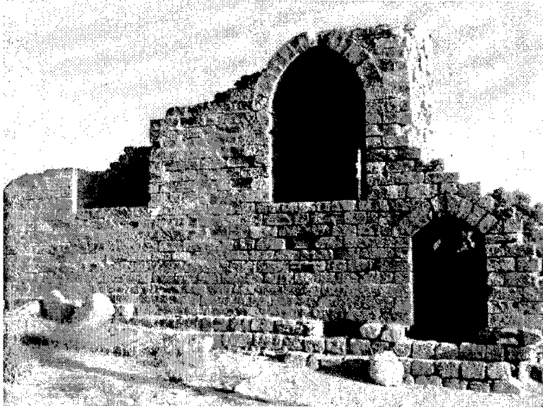
Figure 7. Partially Preserved Section of South Wall. (View south, interior face). Sultan Baybars destroyed Caesarea's walls in 1265 CE, leaving few sections standing above 1.5 meters. This section in the south wall is preserved to a height of nine out of an original ten meters. The arched openings are defensive positions, loopholes, providing access to arrow slits.
