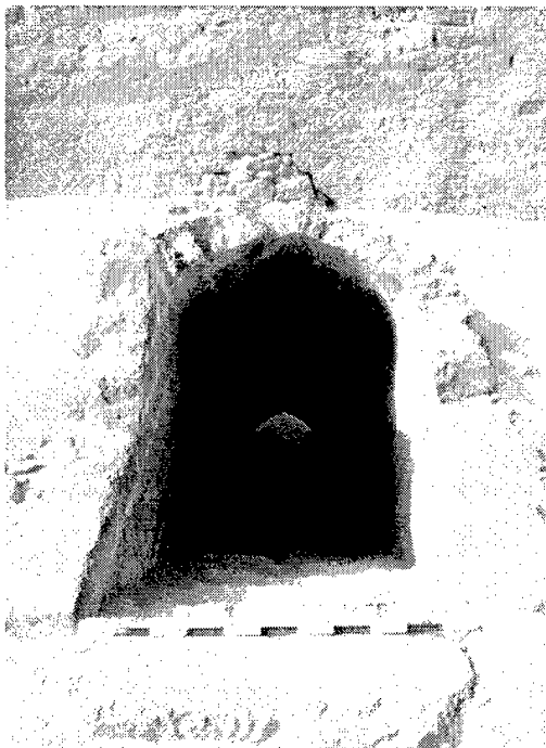
Figure 30. South Postern Top Entrance. (View south, interior south wall). Opening measures approximately one meter wide.
