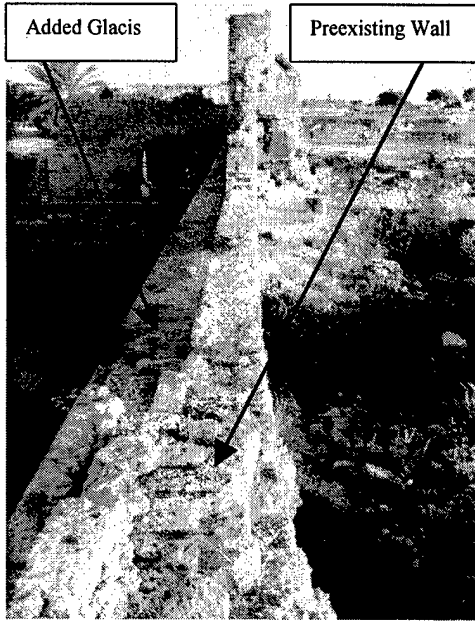
Figure 19. Crusader Phasing in Curtain Wall at East Gatehouse. (View south, profile). Louis IX added the gatehouse in 1251, along with the ashlar exterior facing (glacis).
