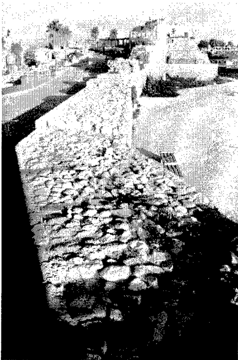
Figure 12. Section of South Wall. (View east from area near citadel). Foundation of this wall follows line of Byzantine breakwater.
