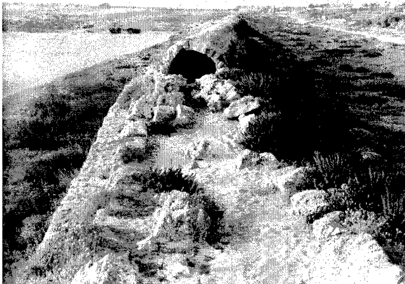
Figure 62. Low-Level Aqueduct. (View north, 150 meters east of the shore line). Although now filled in with sand, the low-level aqueduct had a vaulted channel 2.2 meters high. Probably constructed in the Byzantine period to provide water for agricultural use. Muslims gained access to Caesarea and conquered the city in 640 CE through this water channel.
