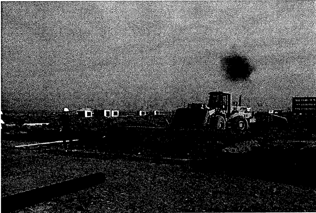
Photograph 5.3: Placing and Leveling Soil for Lift #1
