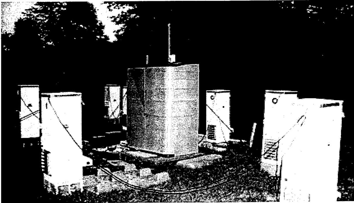
**Figure 2.4.** Electronic hives at Churchville Reference Site, 1997. Each of the “condo” hives contains a mini-hive with a colony of bees. The small storage shed houses a bank of three computers. The weather station mast can be seen extending above the roof of the shed.
