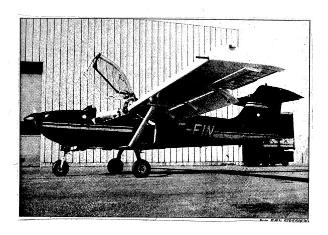
The first airplane wing on a Swedish power plane made entirely of glass-fiber and carbon-fiber composites now has been tested in the air. The test was made on an MFI-15 on which the usual wings were replaced with new wings by a team in Malmo under the leadership of the "father of the MFI," Rudolf Abelin.
