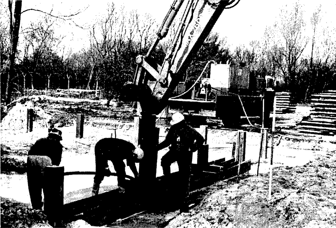
Figure 3.3 Start of the construction of the wooden box. First, some wooden piles are driven into the ground. The piles are used as a framework to strengthen the construction of the walls.
