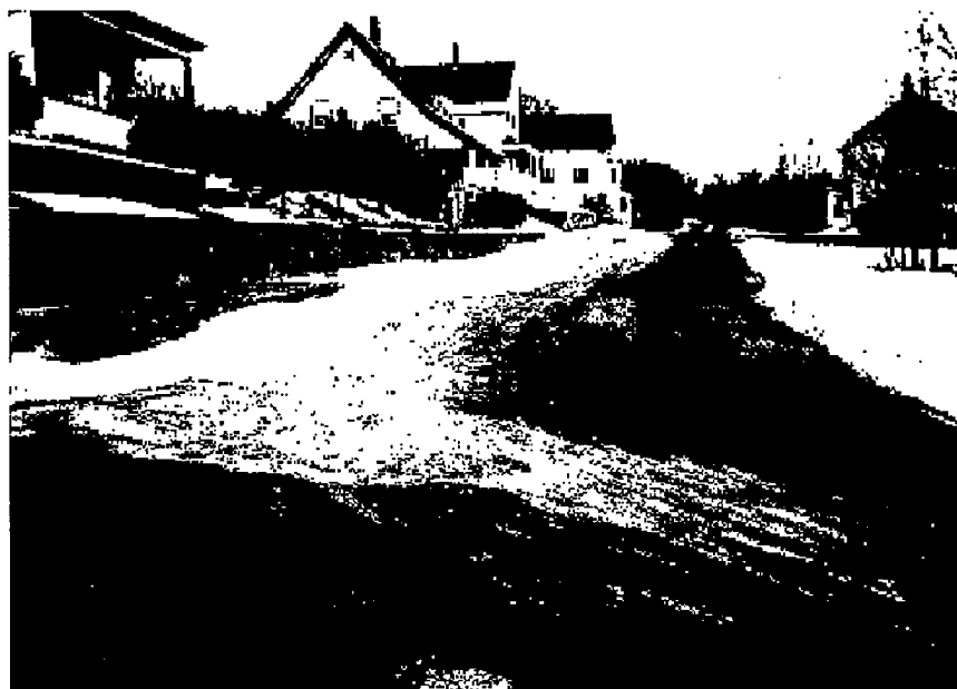
Figure 17. Wentworth Street showing clear roadway over insulated pipeline while rest of road has light snow cover.
