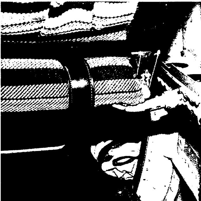
FIGURE 33. STANDARD BEEHCRAFT SEAT (BROWN), AFTER IMPACT
