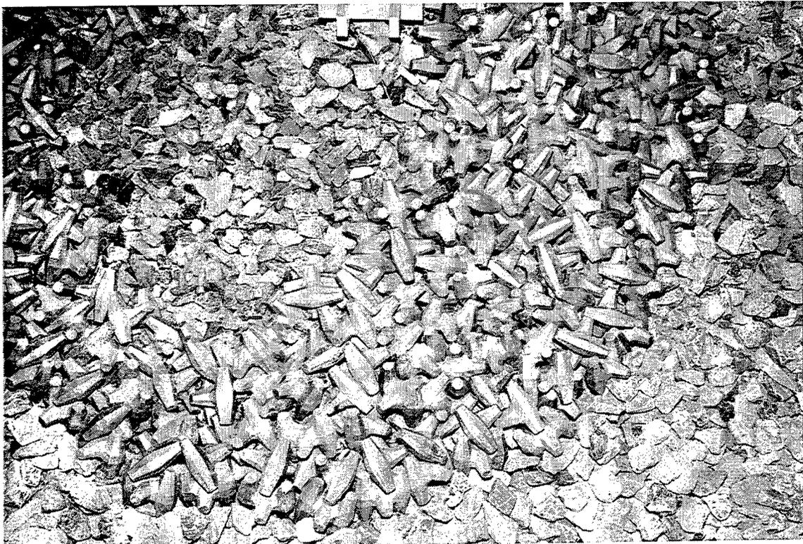
Figure 58. Placement of core-locs
