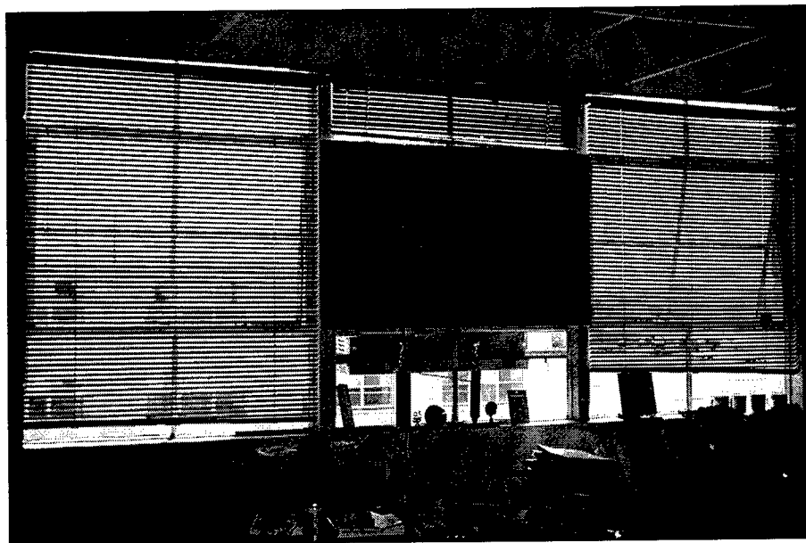
Figure 13. Venetian blinds on windows retard sunlight from entering the Natural Resource director's office where cultural resource records are stored.
