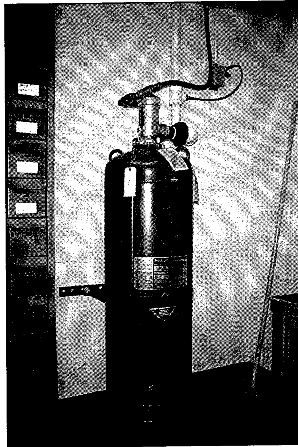
Figure 9. Large halon tank in the collections storage room in Building 156.
