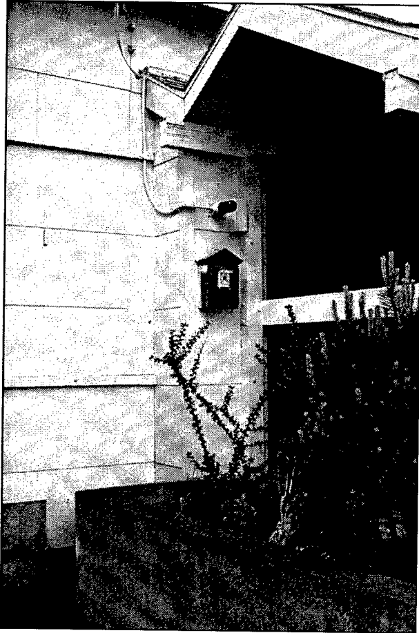
Figure 20. A manual fire alarm is located near an exterior door of Building 119.
