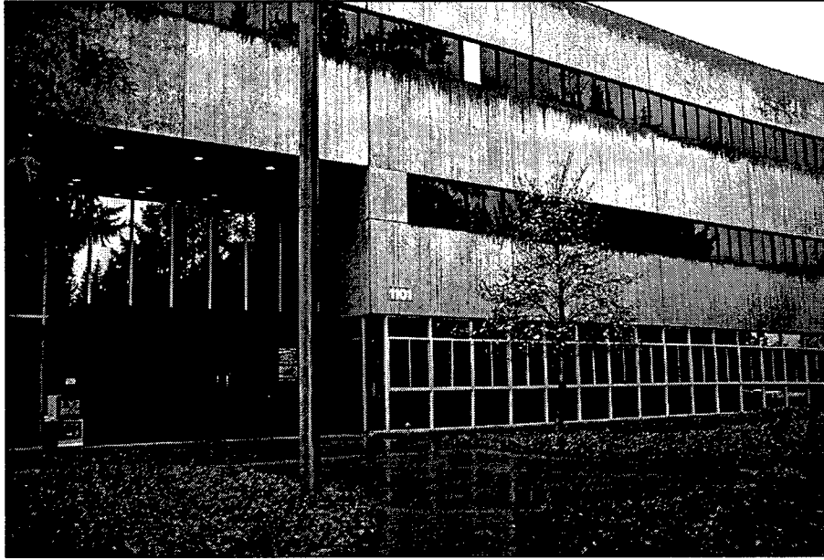
Figure 29. The Public Works Department offices for SUBASE Bangor are housed in Building 1101.
