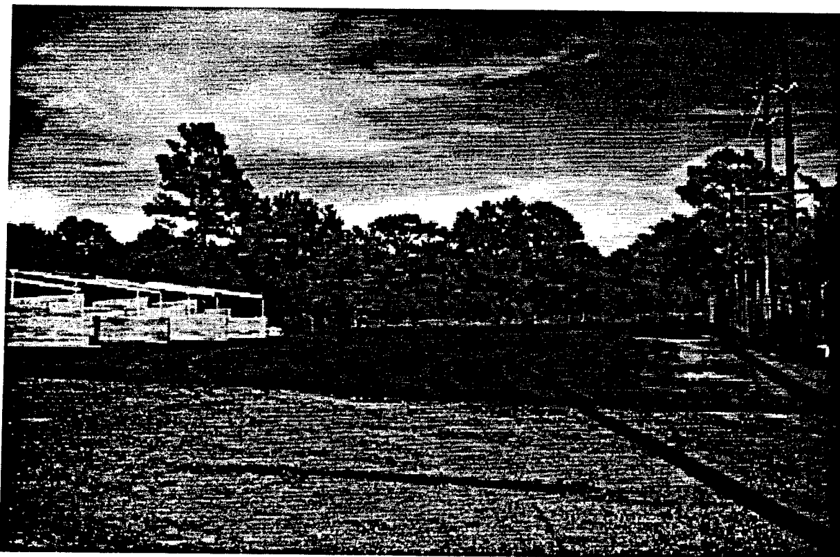
Figure 5. Asphalt pad with bermed sides built to house the vendors' plants. The pad was graded into a containment pond at the far end. Processed soil storage bins are on the left, and pole transformers are on the right.
