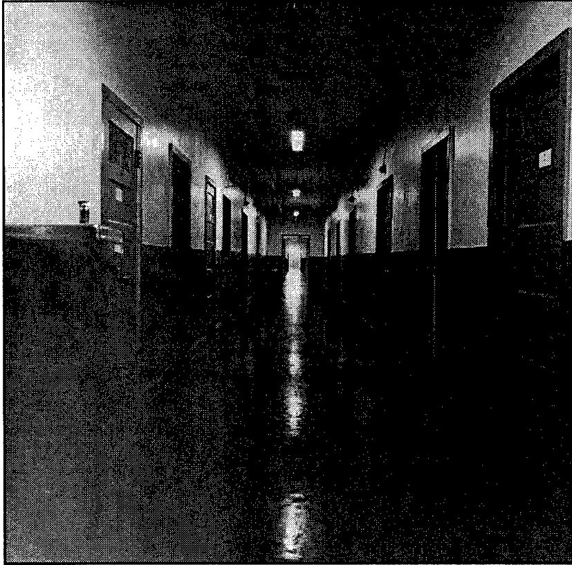
Figure 12. Interior view of a special-ward second-floor hallway (Building S6262). Note the call lights over the doorways to the patients' rooms.
