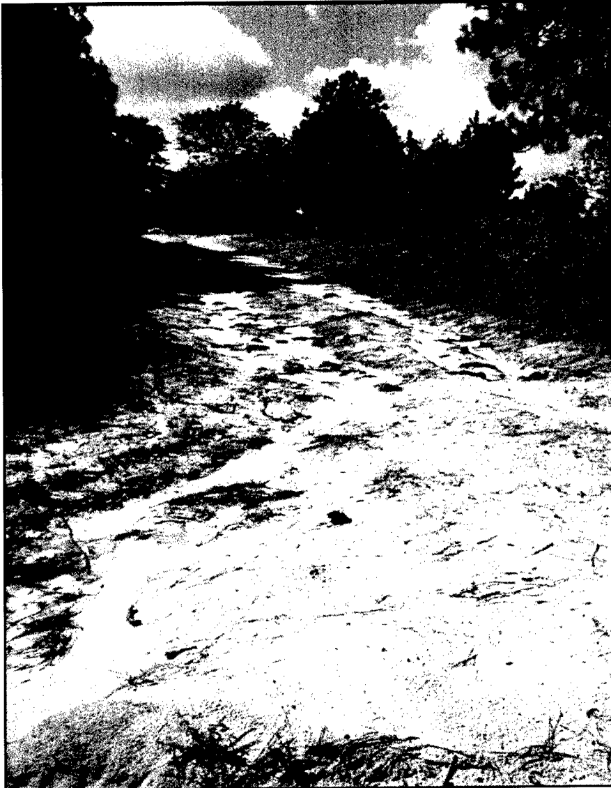
Figure 15. Erosion on sandy, sloped soils usually leads to gully erosion.
