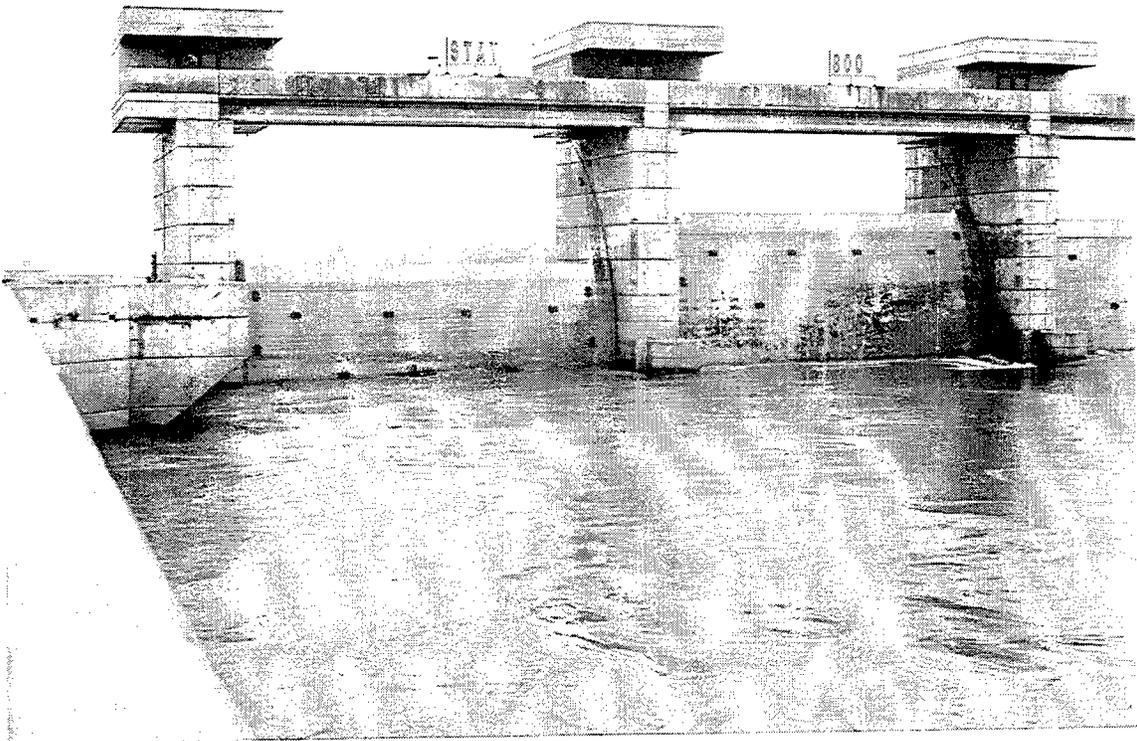
b. Spillway (Gate 1 open 10 ft; Gates 2-5 open 22 ft), 29 Jan 1991
