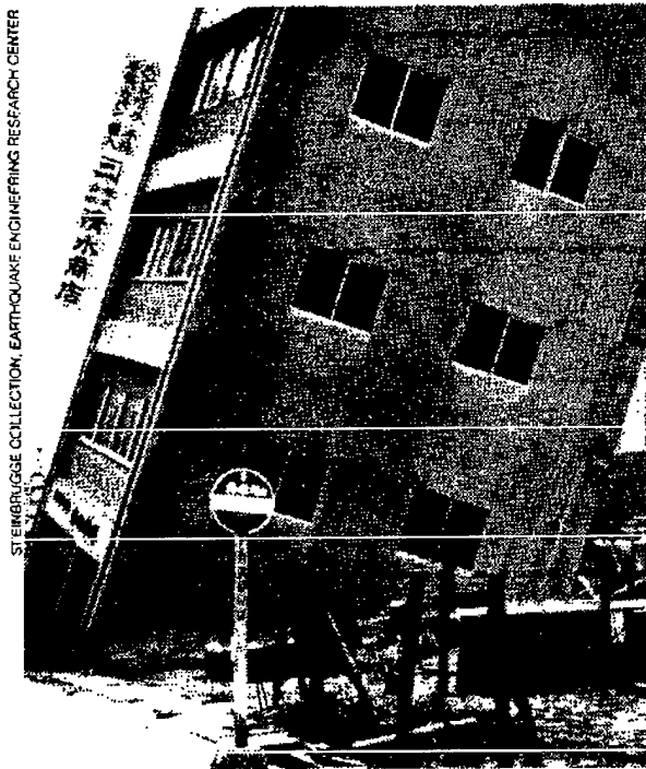
Failure of the ground itself can make an otherwise sound building unusable.
