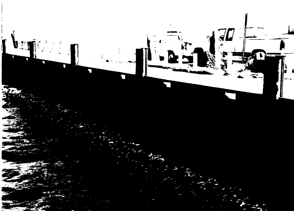
View of steel and timber sheet pile bulkhead along east side of the harbor.
